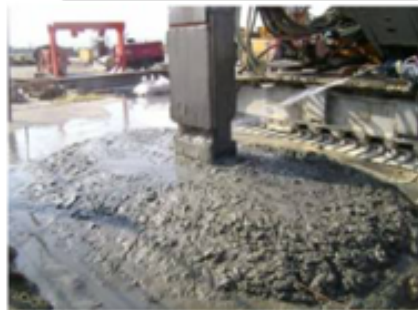
Slurry wall Excess material = 100% of treated volume
