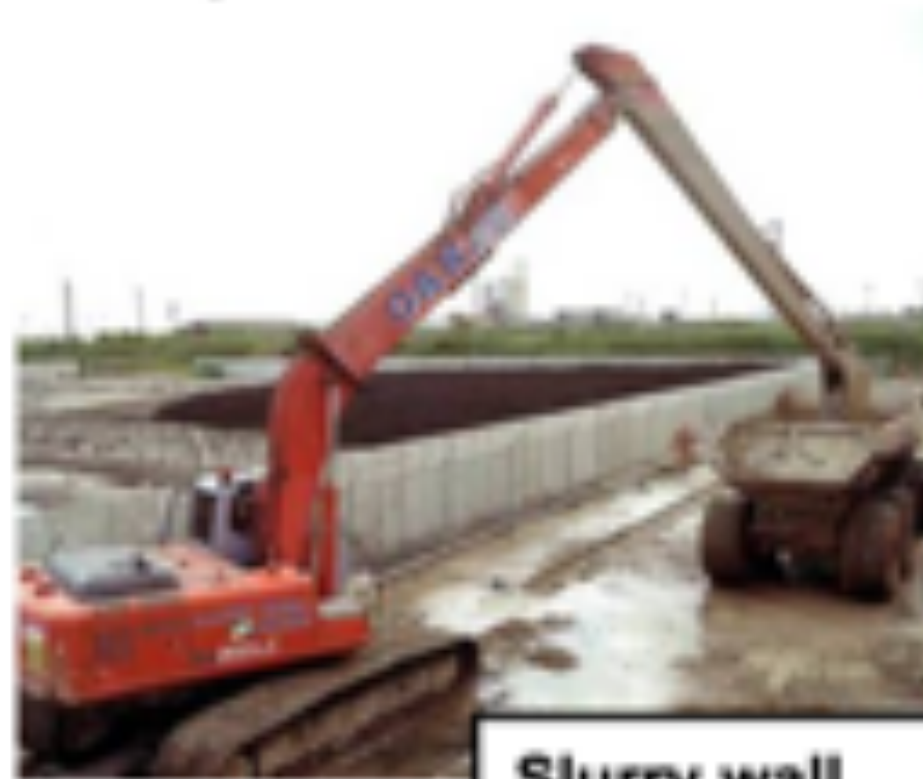
Slurry wall Excess material = 100% of treated volume
