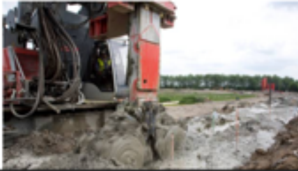
Geomix Excess material < 30% of treated volume
