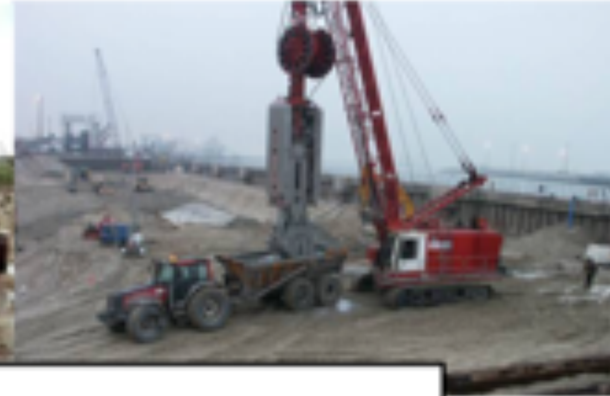
Slurry wall Excess material = 100% of treated volume
