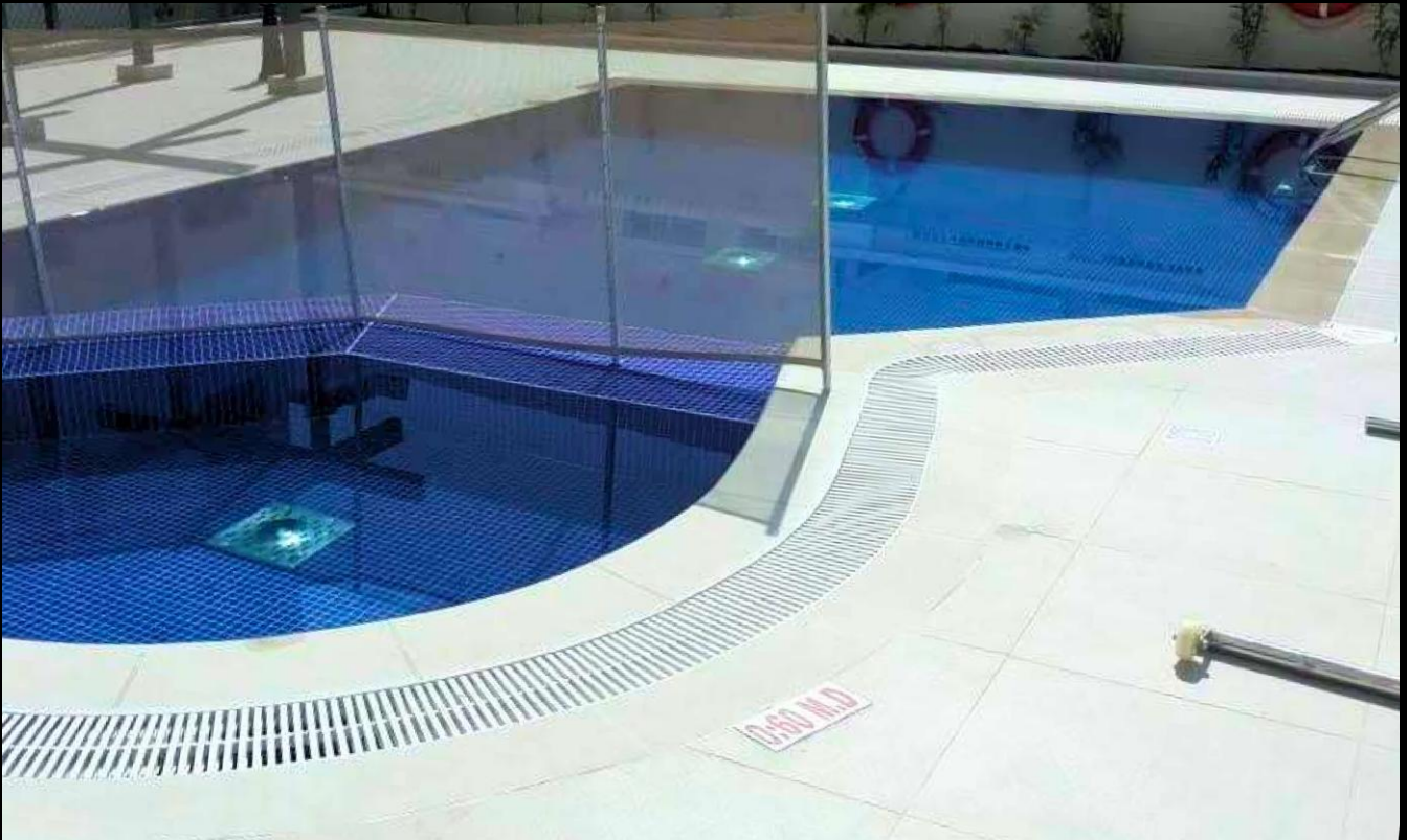
TYPE: Commercial Rooftop Pool - Overflow pool SIZE: 7 X 4 size main pool and 2 X 2 kids pool size
