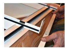
Glue the roof covering as high as possible on the wooden upstand.
