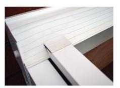
Seal the skylight further with silicone on the wall and the cover profiles.
