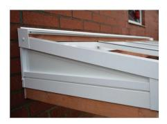
Carefully place the glass with the laminated side on the inside and the coating on the outside in the compartments. The profile on the glass must sit over the cover profile at the bottom. Make sure that all rubbers remain in place.
