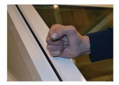
Spray silicone on top of the cover profiles and glue the cover caps on.
