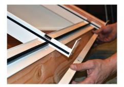
Place the skylight over the roof opening and secure it to the roof every 30cm.
