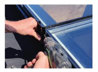
Screw the pressure slats left and right, and if intermediate beams also in the middle, into the ledge of the roof beams, the correct position is indicated on the profiles. These must fit perfectly against the cover plates.
