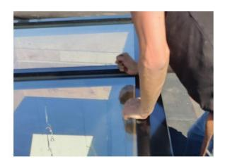
Glue the two corner caps at the top left and right with the supplied silicone.
