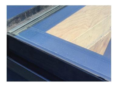
13. Seal the skylight further with silicone at the end pieces. (\*) Intermediate beams
