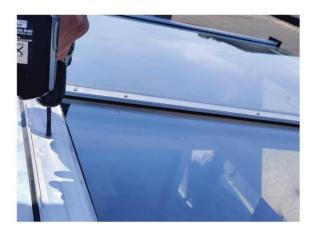
Tap the cover caps left and right, and if intermediate beam(s) in the middle, onto the pressure slats. These must fit perfectly against the cover plates at the bottom. Make sure that they click into place everywhere, if necessary use a wooden block and a hammer.
