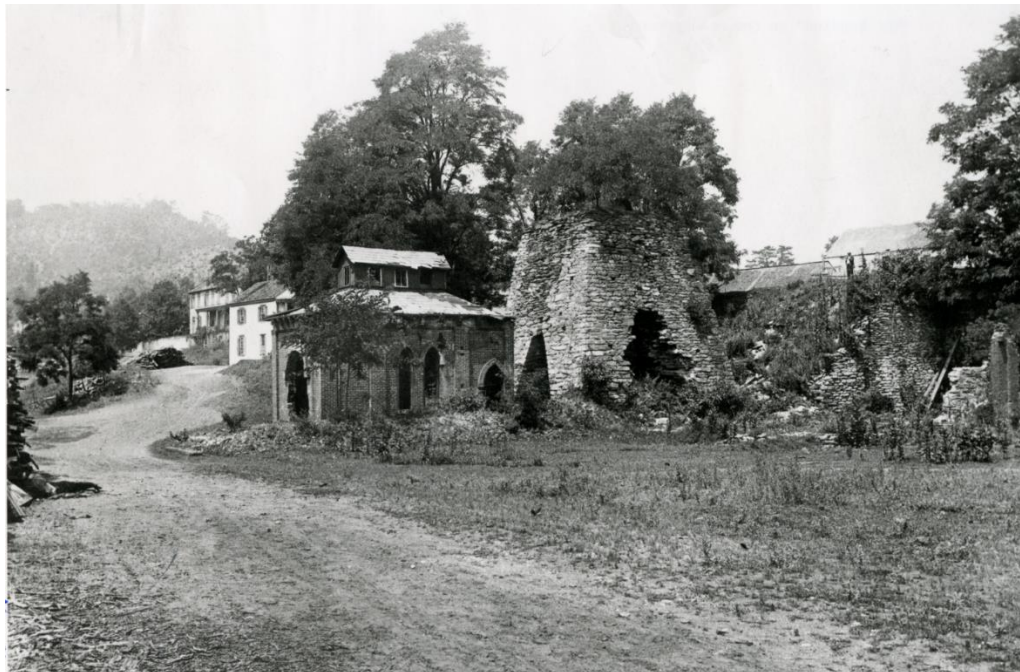
Pine Grove Furnace circa 1914. This photograph was taken after the iron works was purchased by the Commonwealth of Pennsylvania. Note the dilapidated condition of the stone stack, and the removal of most adjoining structures. The Ironmaster's Mansion (far left) and Paymaster's Office (left) are barely visible in the rear of the image.
