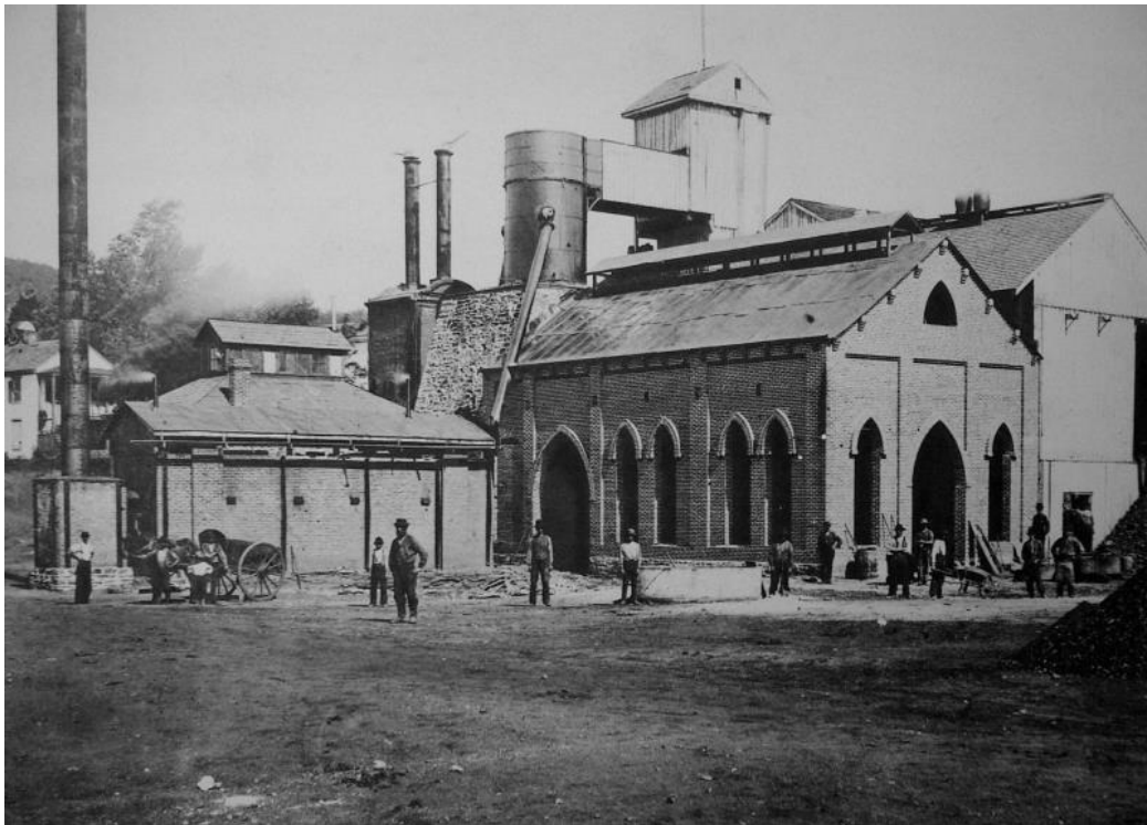
Pine Grove Furnace in the late 19 th century. This view reflects industrial improvements made by engineer John Birkinbine. The top of the stone furnace stack is barely visible in the center. The large building with arched openings is the casting house. The smaller building at left housed a steam engine for forcing air “blast” into the bottom of the furnace.
