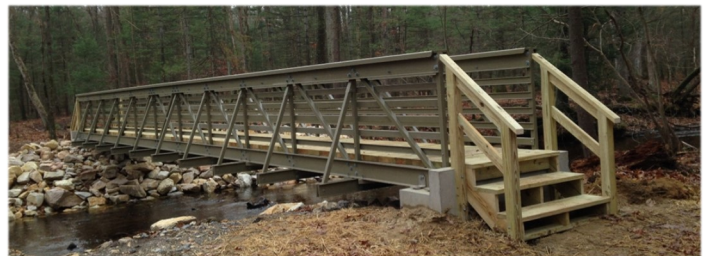
The new hiking bridge across Mountain Creek
