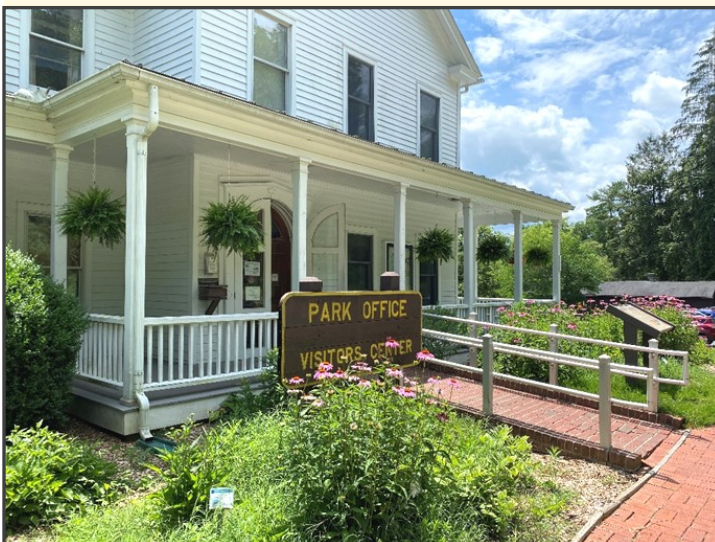
The Park Office was an 1850s boarding house and later a public inn
