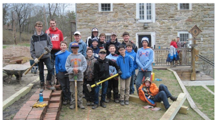
Scouts from Troop 430 at work on the AT Museum walkway
