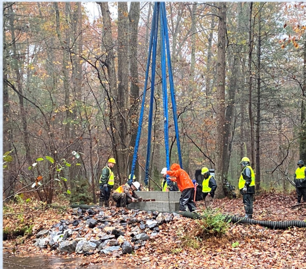
Positioning the abutment for the Koppenhaver Trail side
