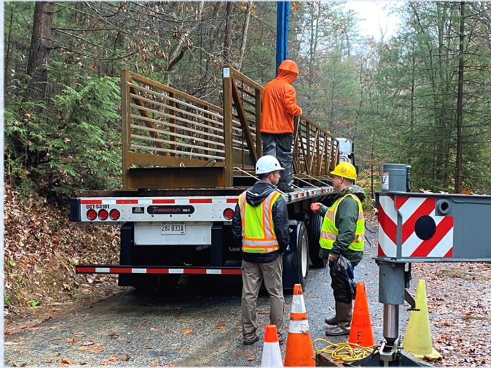
The 50-foot, 5-ton bridge arrived on a flatbed tractor trailer
