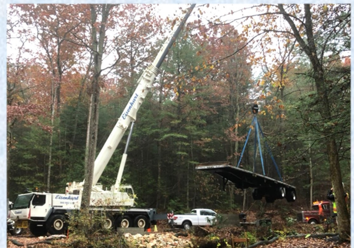
The trailers that carried in the abutments and the bridge were lifted into the air using the crane and turned around for the trip back down the narrow Old Railroad Bed Road
