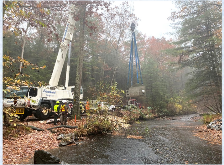
Crane lifting a concrete abutment across Mountain Creek
