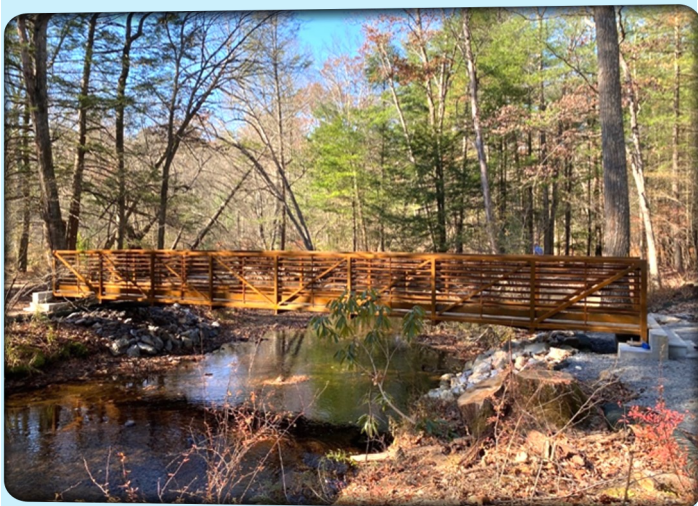
The new connector bridge in early November
