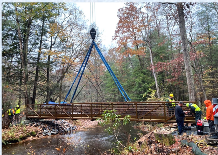
Bolting the bridge into place on the abutments
