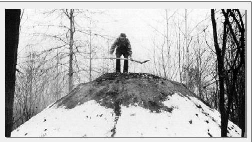
A collier demonstrates "jumping the pit" to push down hollow areas forming inside the huge mound of wood as it slowly smolders into charcoal. Note that he is holding his shovel sideways as a self-rescue tool, just in case he falls into the dangerously hot pit.
