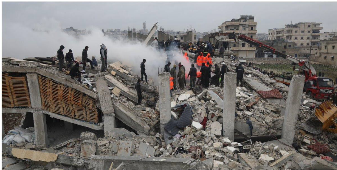
Collapsed building in Sarmada, north-west Syria. 6 February 2023. Credit: OCHA/Ali Haj Suleiman
