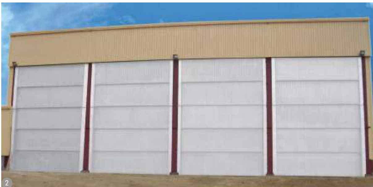
1/ BEN SLIMANE AIRPORT, MOROCCO. 10-LEAF SLIDING DOOR MEASURING 50-M LONG BY 15-M HIGH. 2/ GOLD MINES, MAURITANIA. FOUR VERTICAL SLIDING DOORS MEASURING 9-M LONG AND 12.5-M HIGH.
