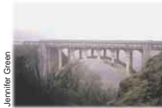
Dry Canyon Bridge
