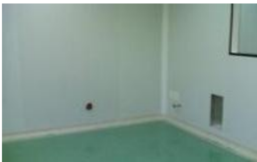
EPOXY COATING FOR OT/CLEAN ROOM
