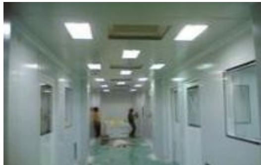
PANELLING TO ICU & WARDS
