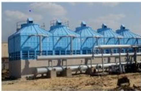
COOLING TOWER INSTALLATION
