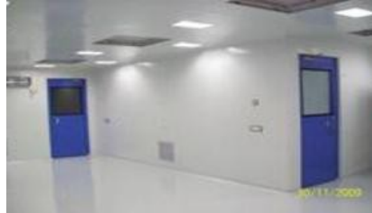
PARTITION PANELLING WITH DOORS & EPOXY
