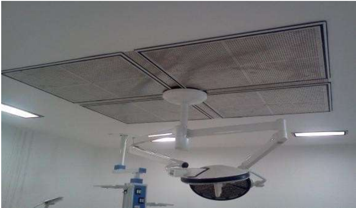
LAMINAR FLOW UNIT NON-ILLUMINATED TYPE WITH SS GRILL, PANEL & COWING
