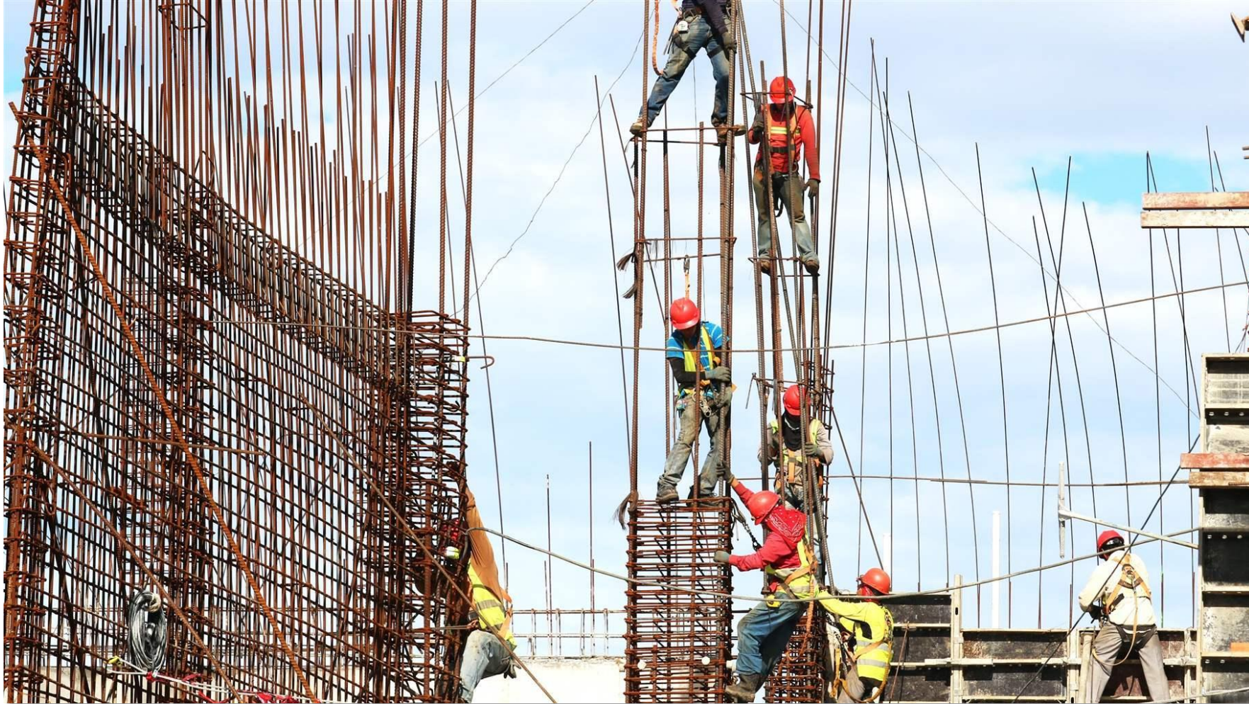
Rebar's Erection
