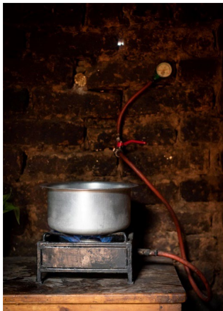
The biogas installation
