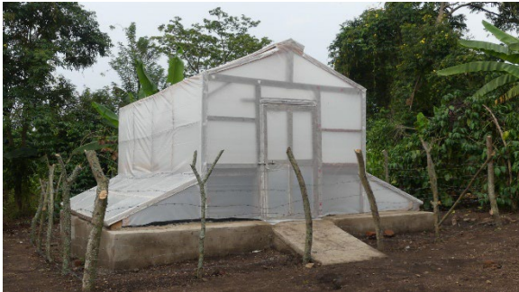
Solar dryers for coffee, maize and fruits
