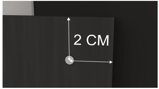
When screwing the plank, it is necessary to observe the specified distances from the edges of the plank, otherwise the edges of the plank may be split.
