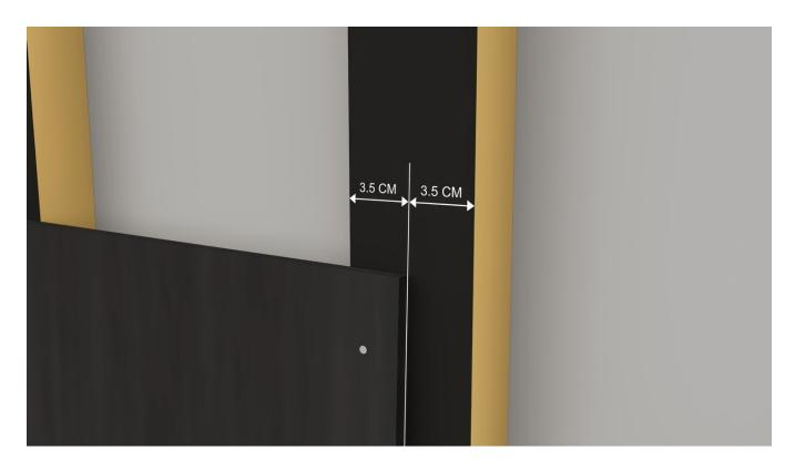
When connecting the panels, it is necessary to connect them on the middle of the frame slats. It is forbidden to screw additional brackets.
