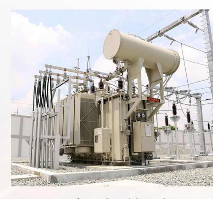
A power transformer is mainly used to transmit high electric power at high voltage levels through power lines to the distribution centers. They generally have high MVA ratings. Power transformers are mainly used for increasing low voltage levels to high voltage levels for transmission, maximizing efficiency at or close to full loads
