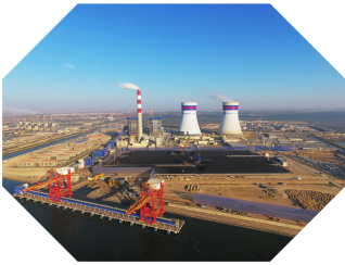
electricity power plant
