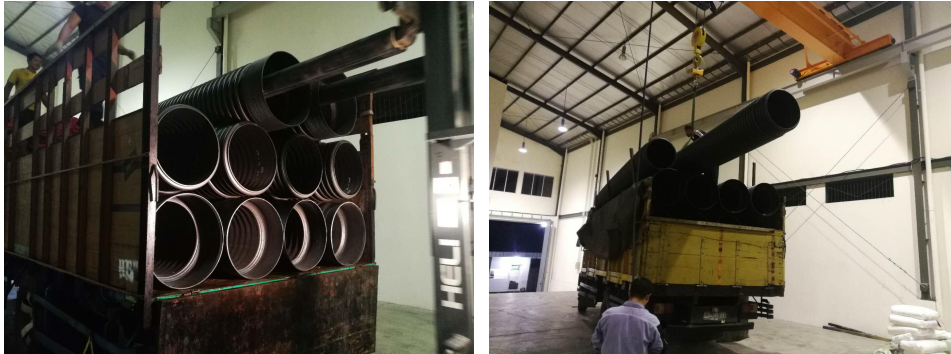
Surabaya projects used HDPE double wall corrugated pipe (ID500mm)
