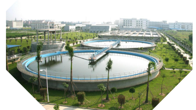
waste water treatment
