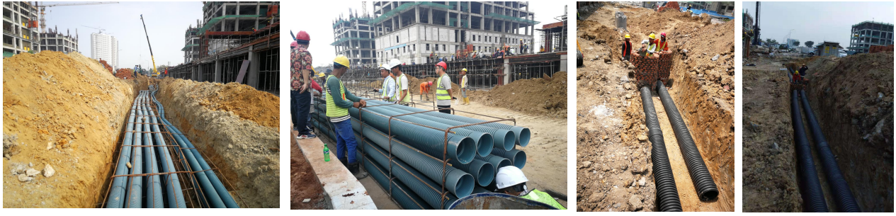
MEIKARTA projects (applied HDPE double wall corrugated pipe)
