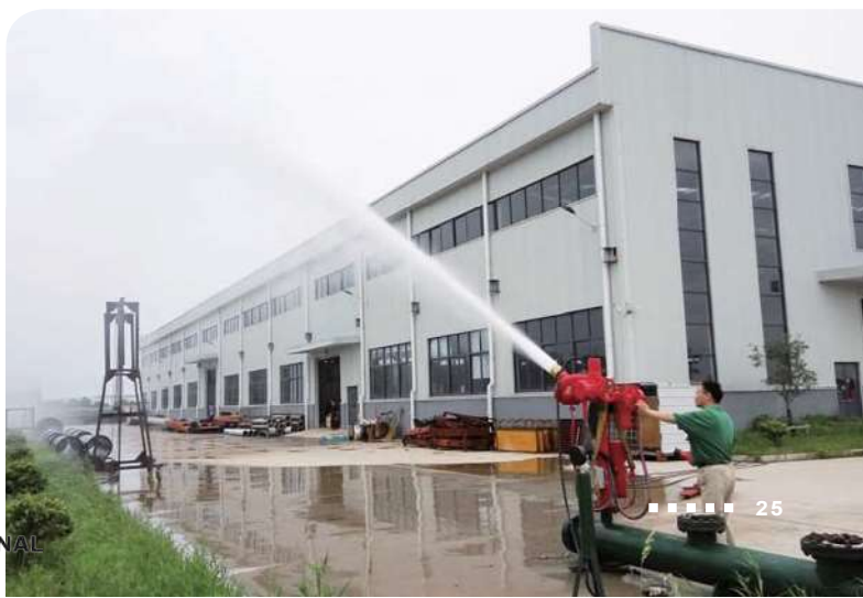
Fire monitor testing area
