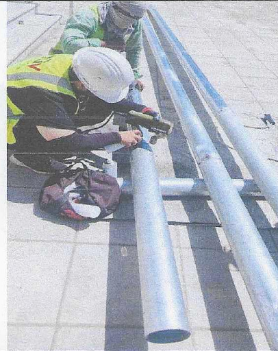
5. Welding joints NDE-MPI 10% were inspected and found satisfactory.
