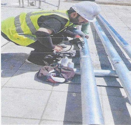
4. Welding joints NDE-MPI 10% were inspected and found satisfactory.
