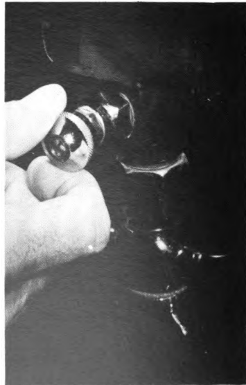
Figure 425.—Closing the water pressure regulator and shutoff valve.
