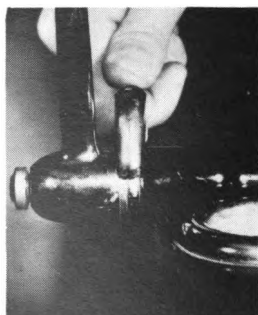
Figure 435.—Tightening the bonnet.
