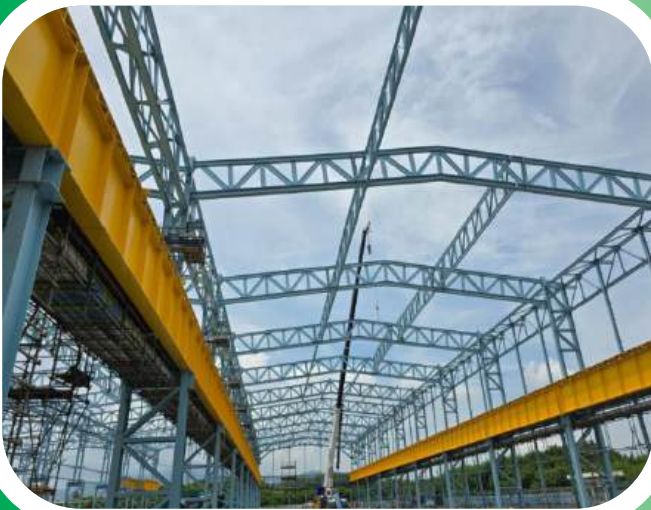
■ Install Longitudinal Truss PT. KRAKATAU POSCO
