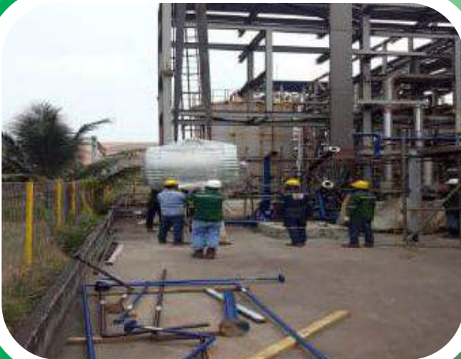
■ Erection Exchanger
