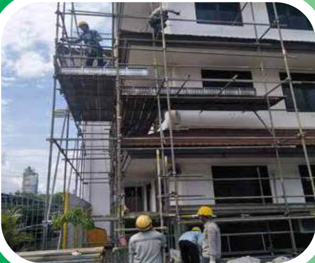
■ Scaffolding Service at Building
