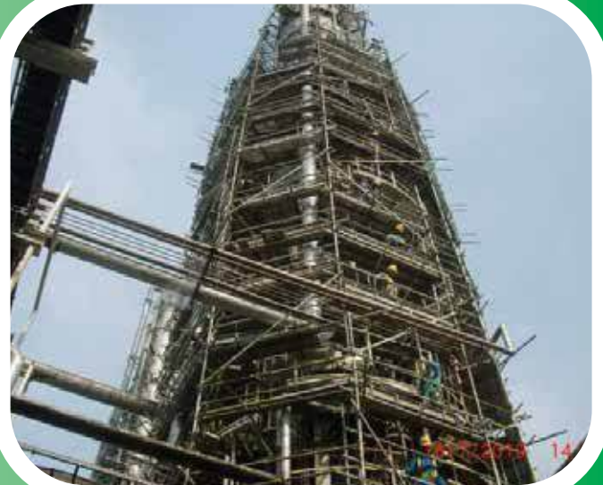
■ scaffolding service at coloum destilation
