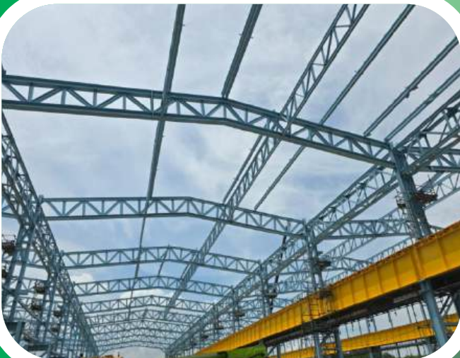
■ Install Purlin Roof PT. KRAKATAU POSCO
