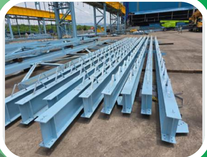
■ Install Connector Roof PT. KRAKATAU POSCO
