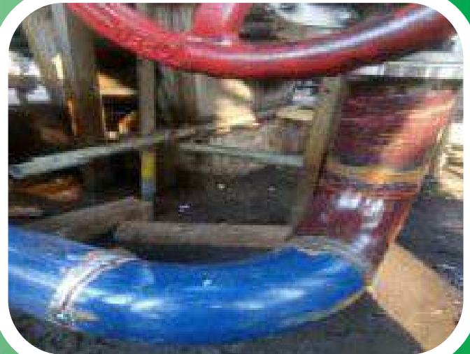
■ Instal Pipe Spool
