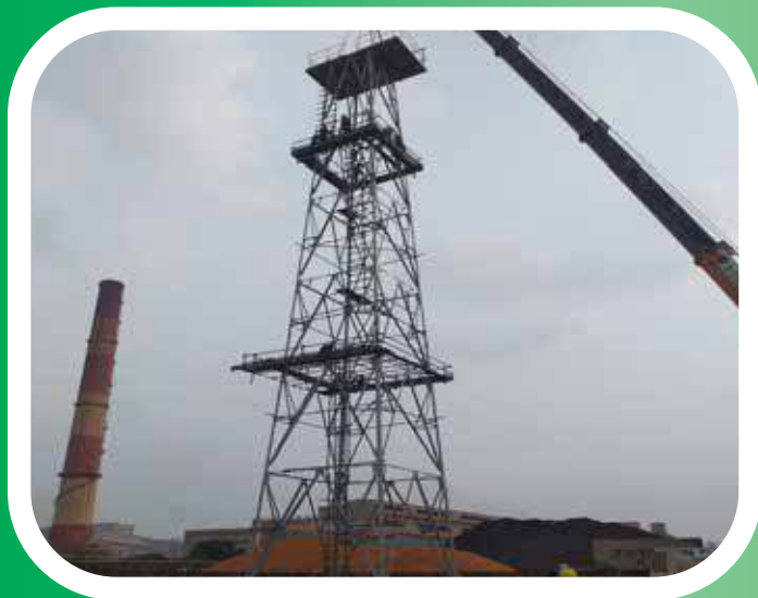
■ Erection Lighting Tower, RMH PT. KRAKATAU POSCO
