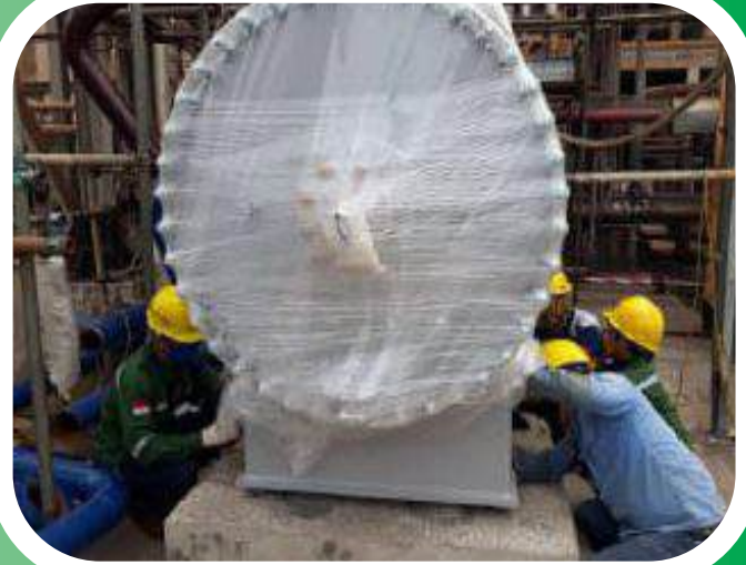
■ Erection Exchanger
