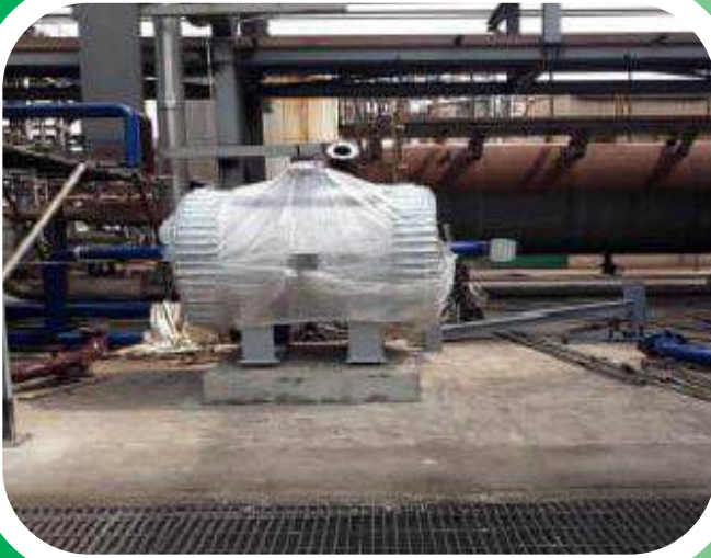
■ Erection Exchanger
