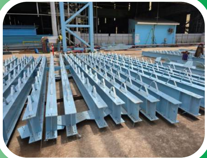
■ Install Connector Roof PT. KRAKATAU POSCO
