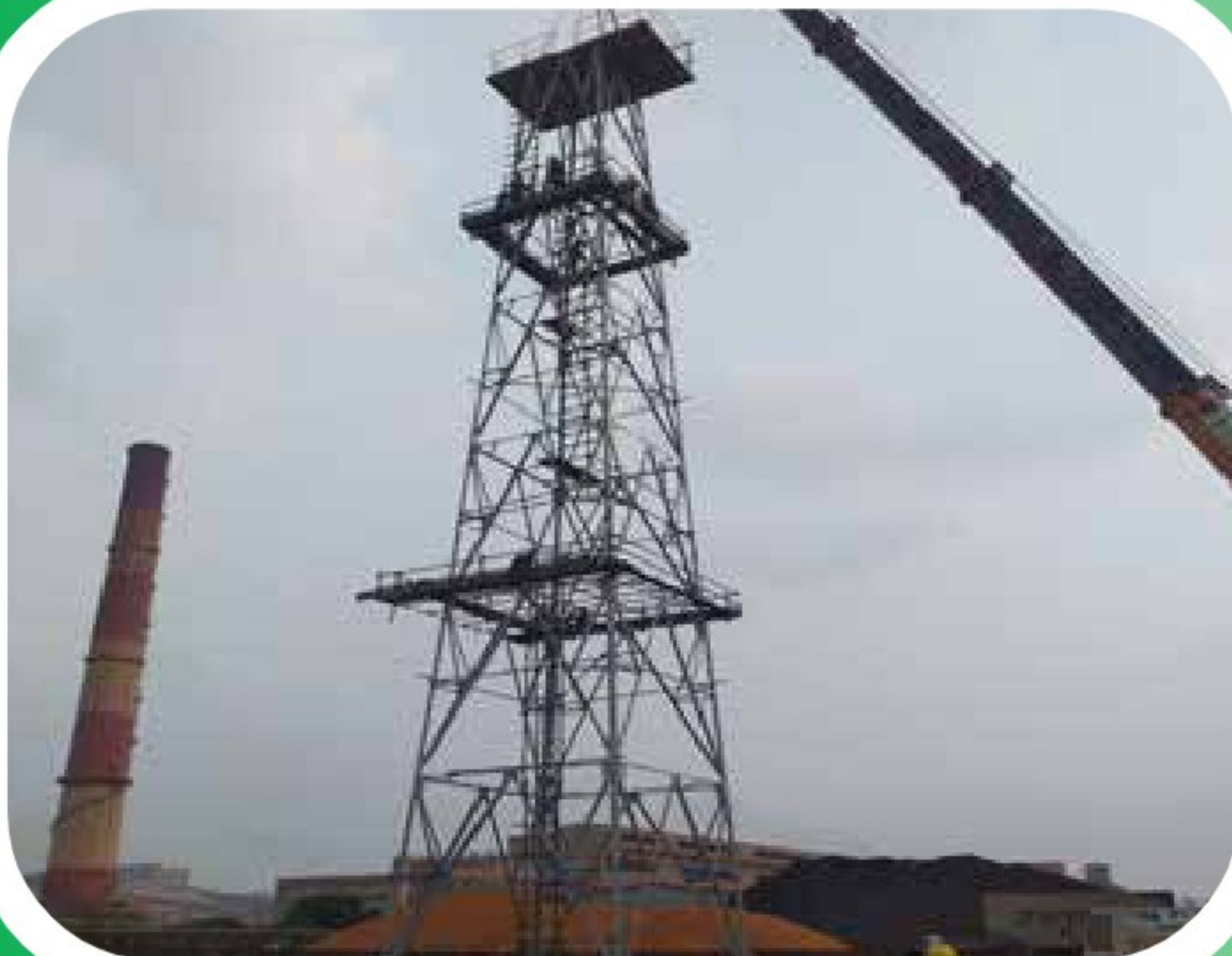
■ Erection Lighting Tower, RMH PT. KRAKATAU POSCO
