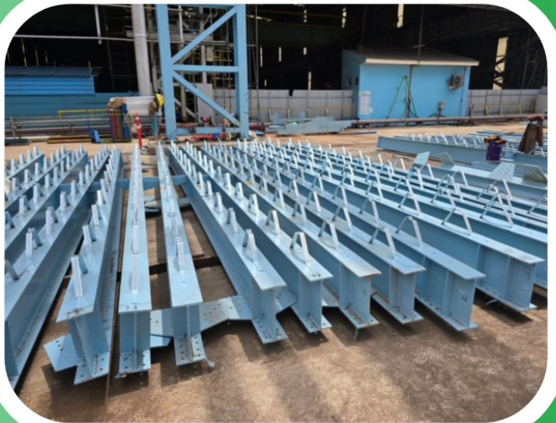
■ Install Connector Roof PT. KRAKATAU POSCO
