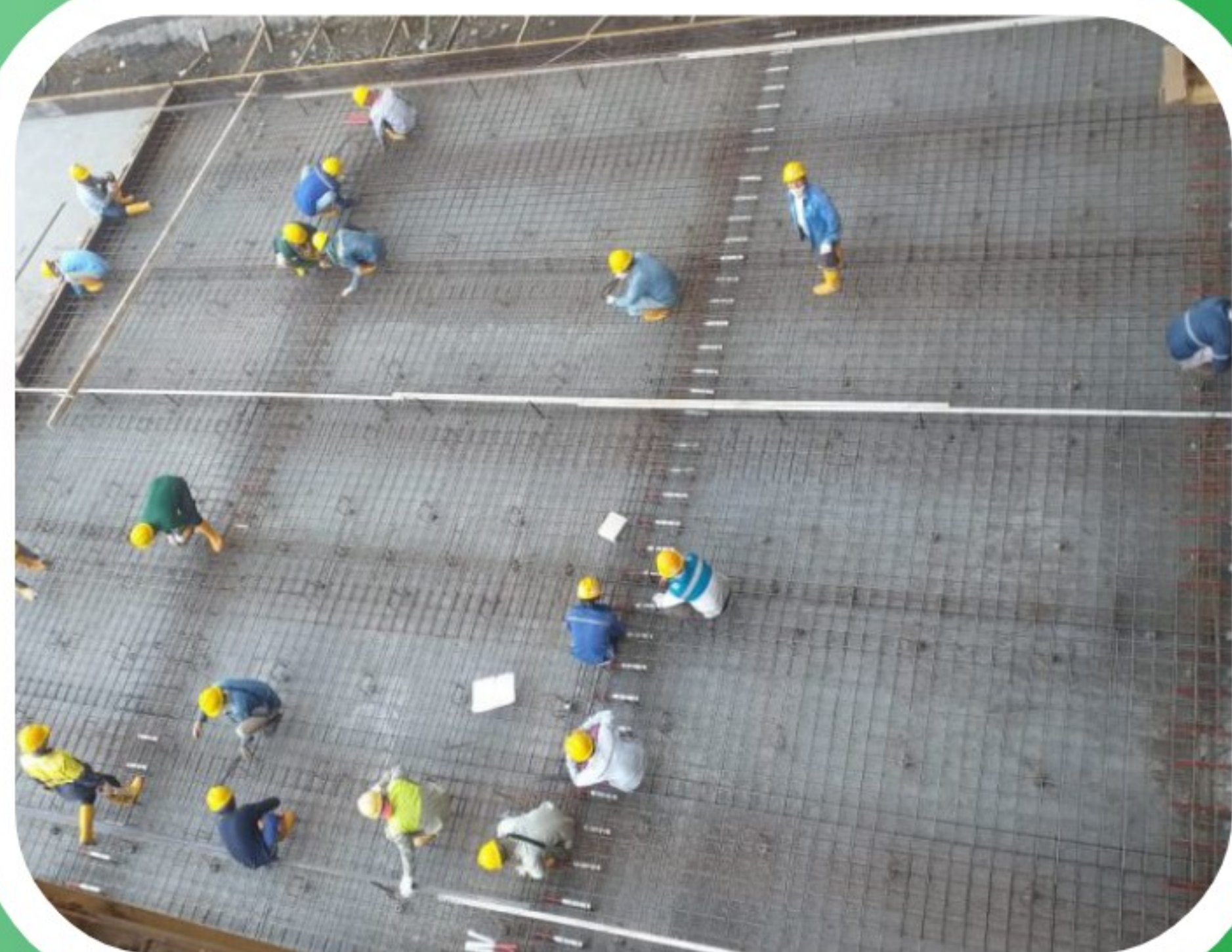
■ Project New Slab Route For New HSM (Package 1) PT. KRAKATAU POSCO
