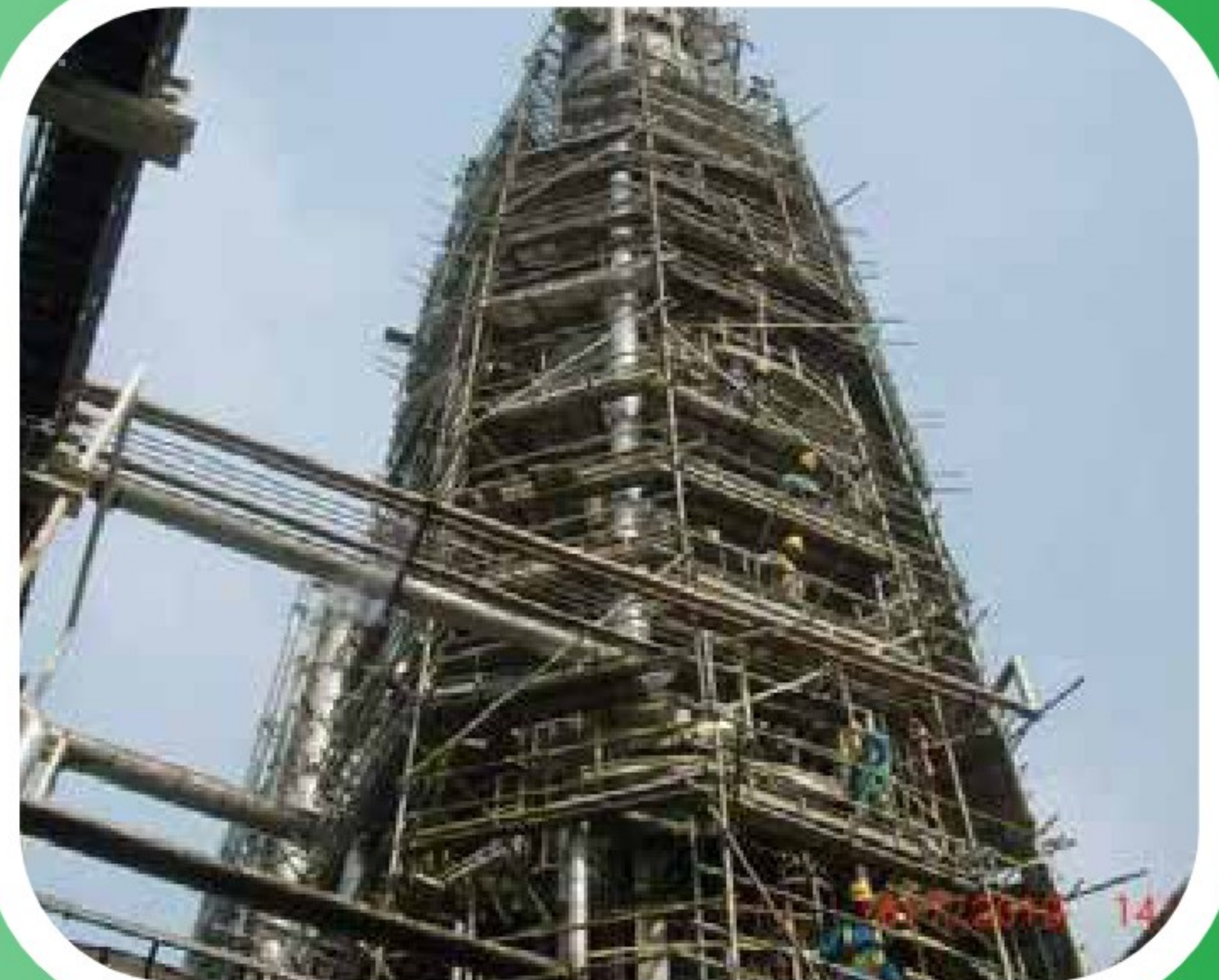
■ scaffolding service at coloum destilation
