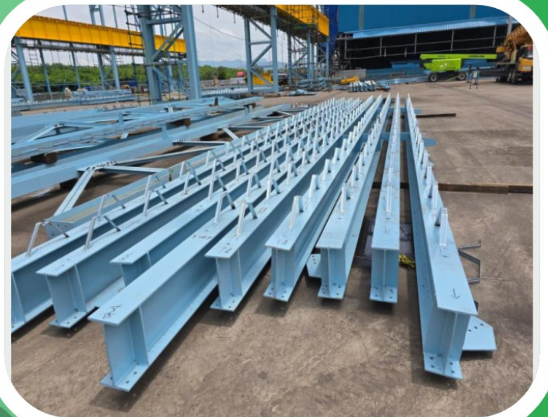
■ Install Connector Roof PT. KRAKATAU POSCO
