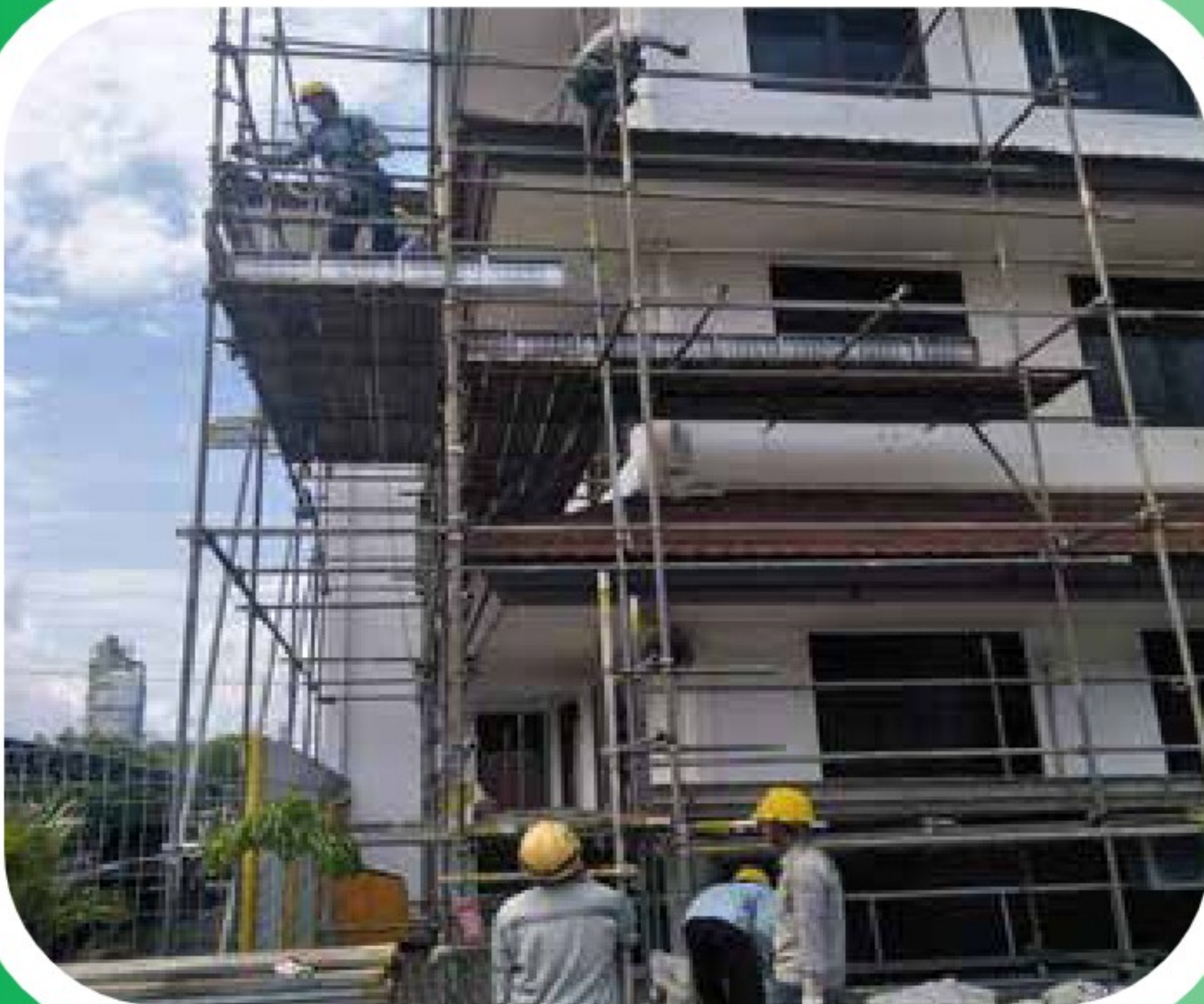
■ Scaffolding Service at Building
