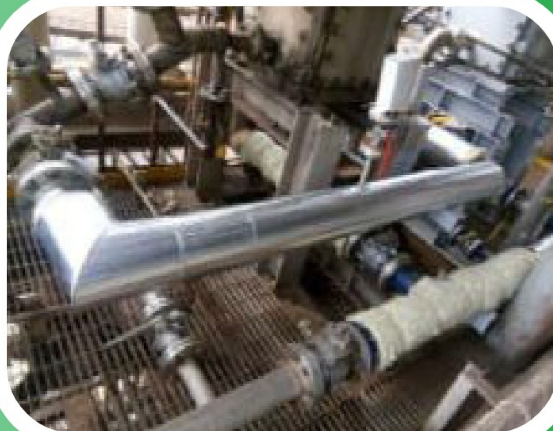
■ BTX Heat Exchanger Installation in Coke for PT. KRAKATAU POSCO
