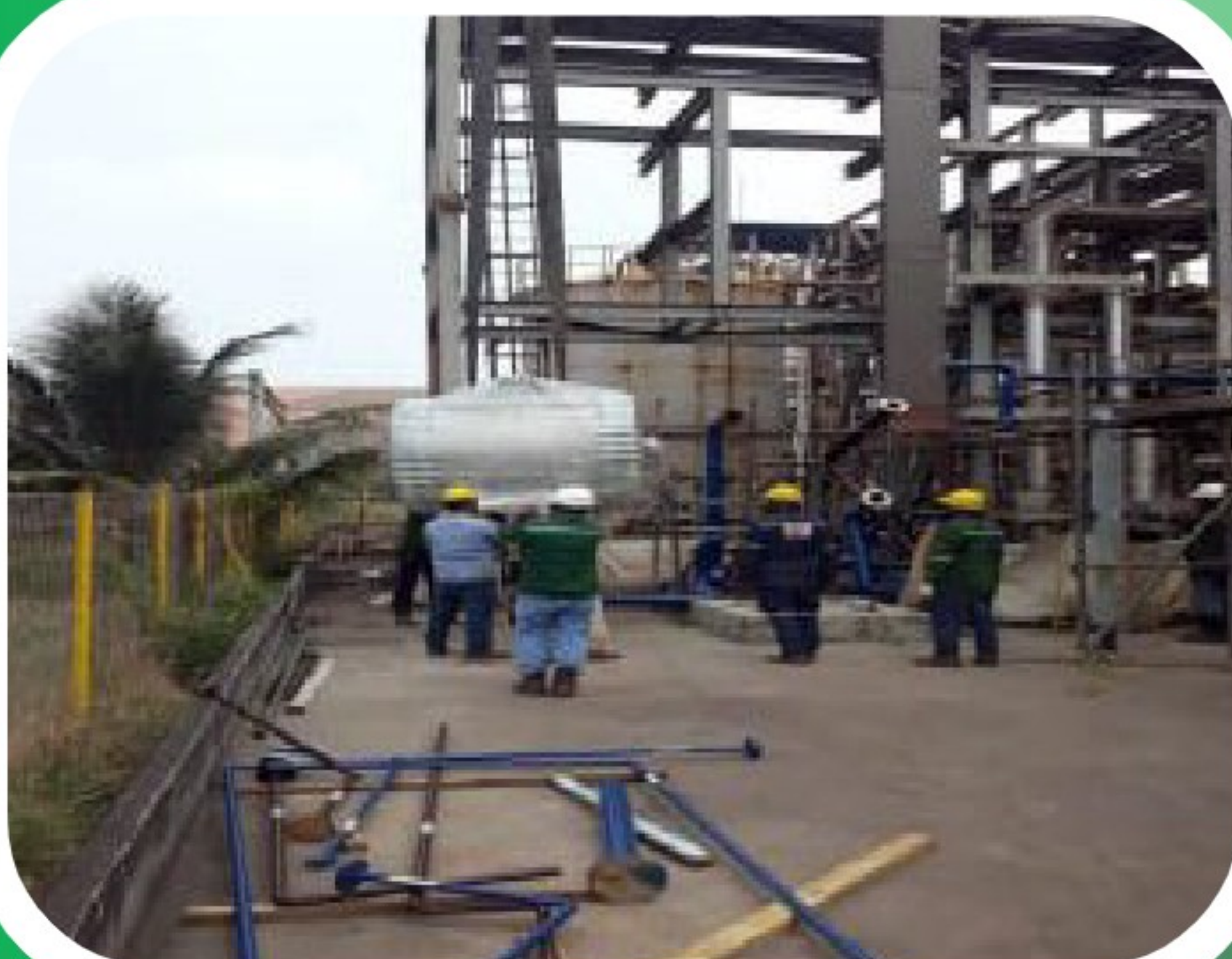
■ Erection Exchanger
