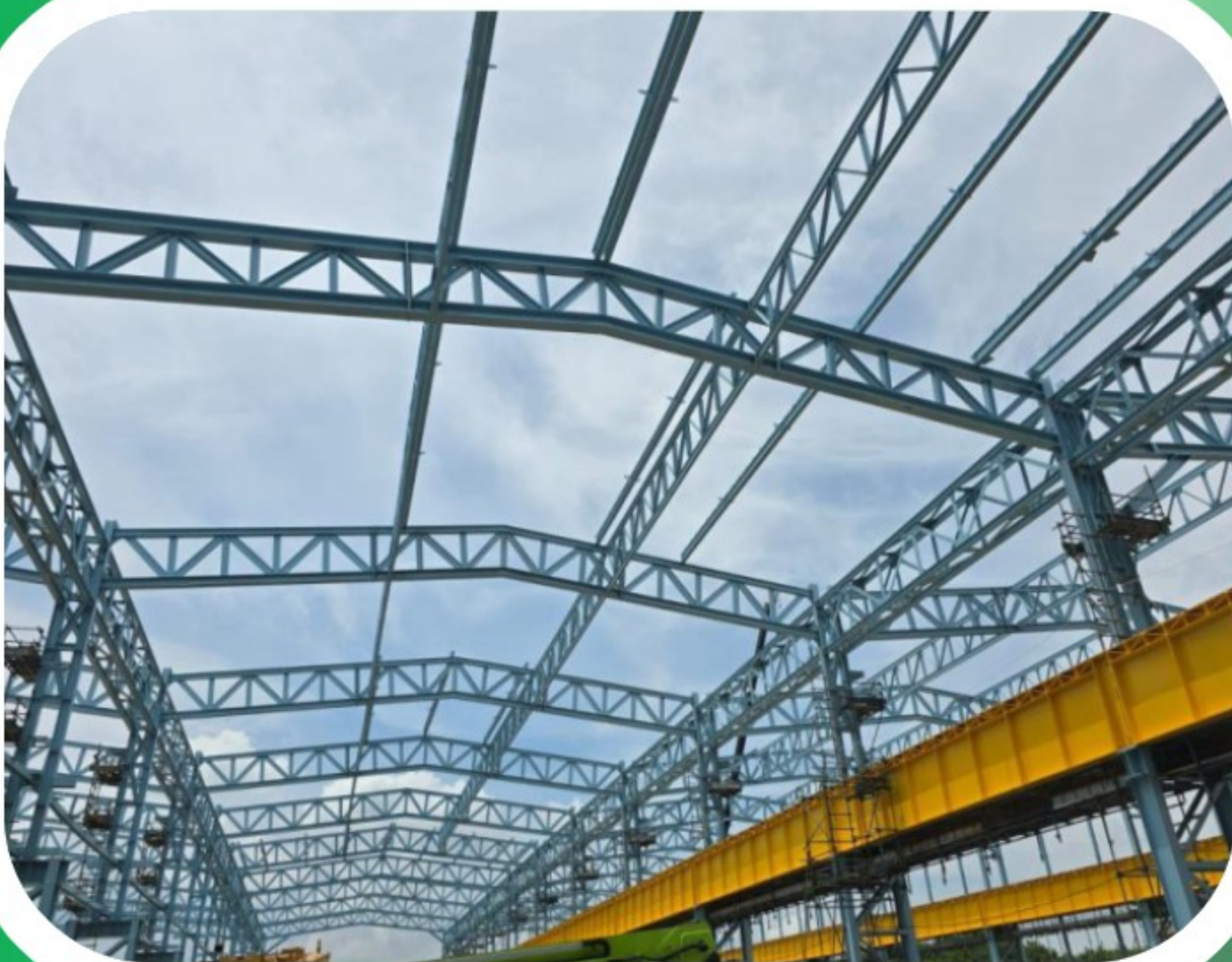
■ Install Purlin Roof PT. KRAKATAU POSCO
