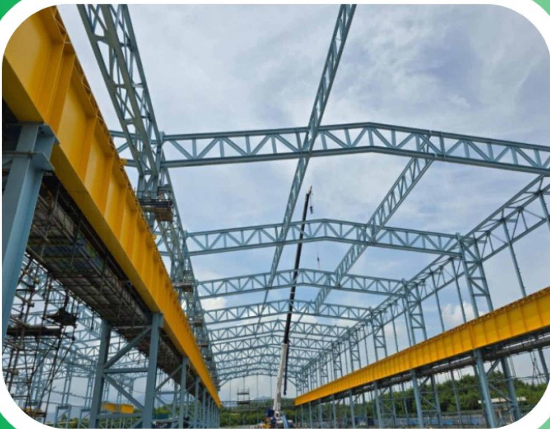
■ Install Longitudinal Truss PT. KRAKATAU POSCO
