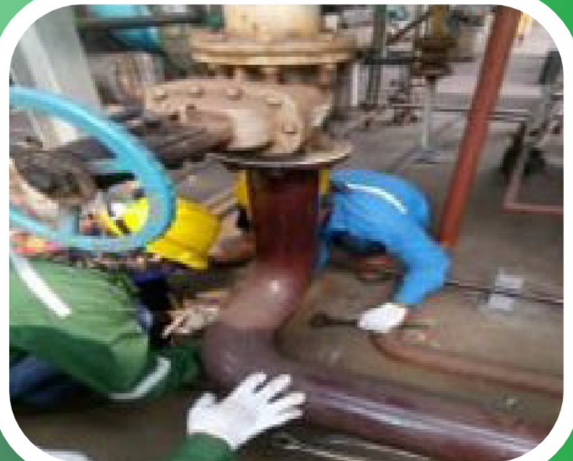
■ BTX Heat Exchanger Installation in Coke for PT. KRAKATAU POSCO
