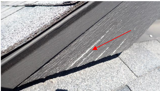
Areas of roofing barge boards.
