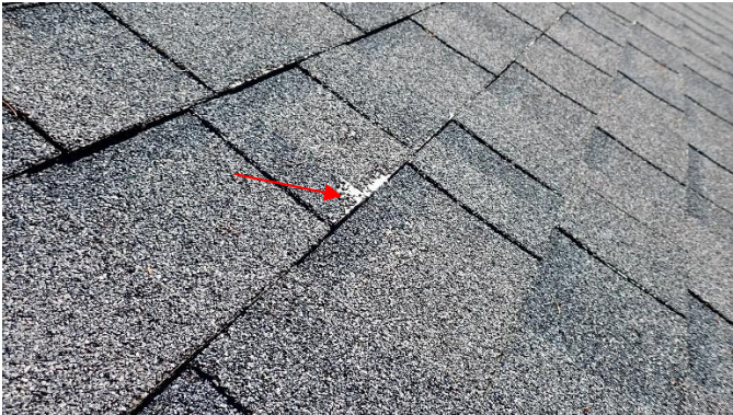
Examples below of exposed fibers along composition edges.
