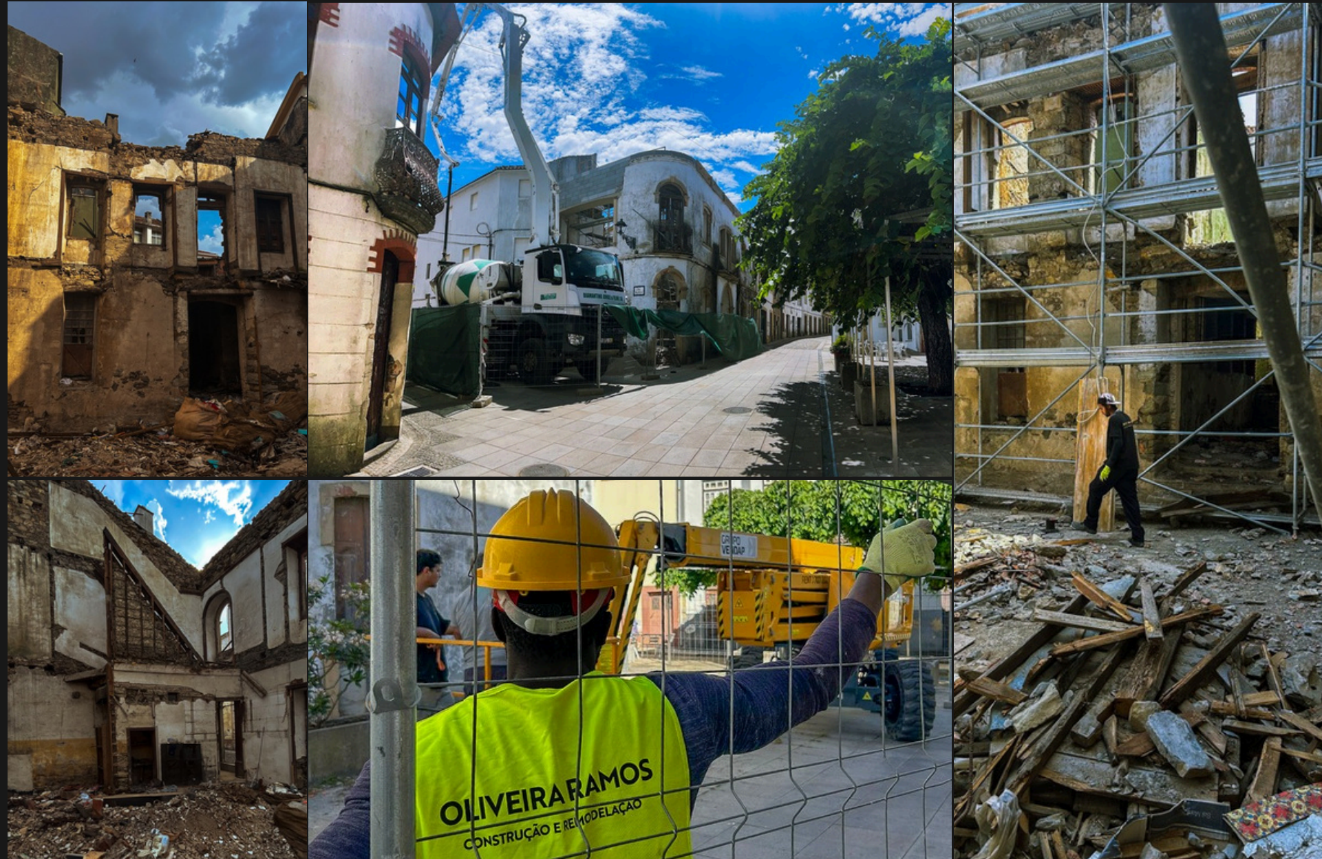
DEMOLITION IN PROENÇA A NOVA
