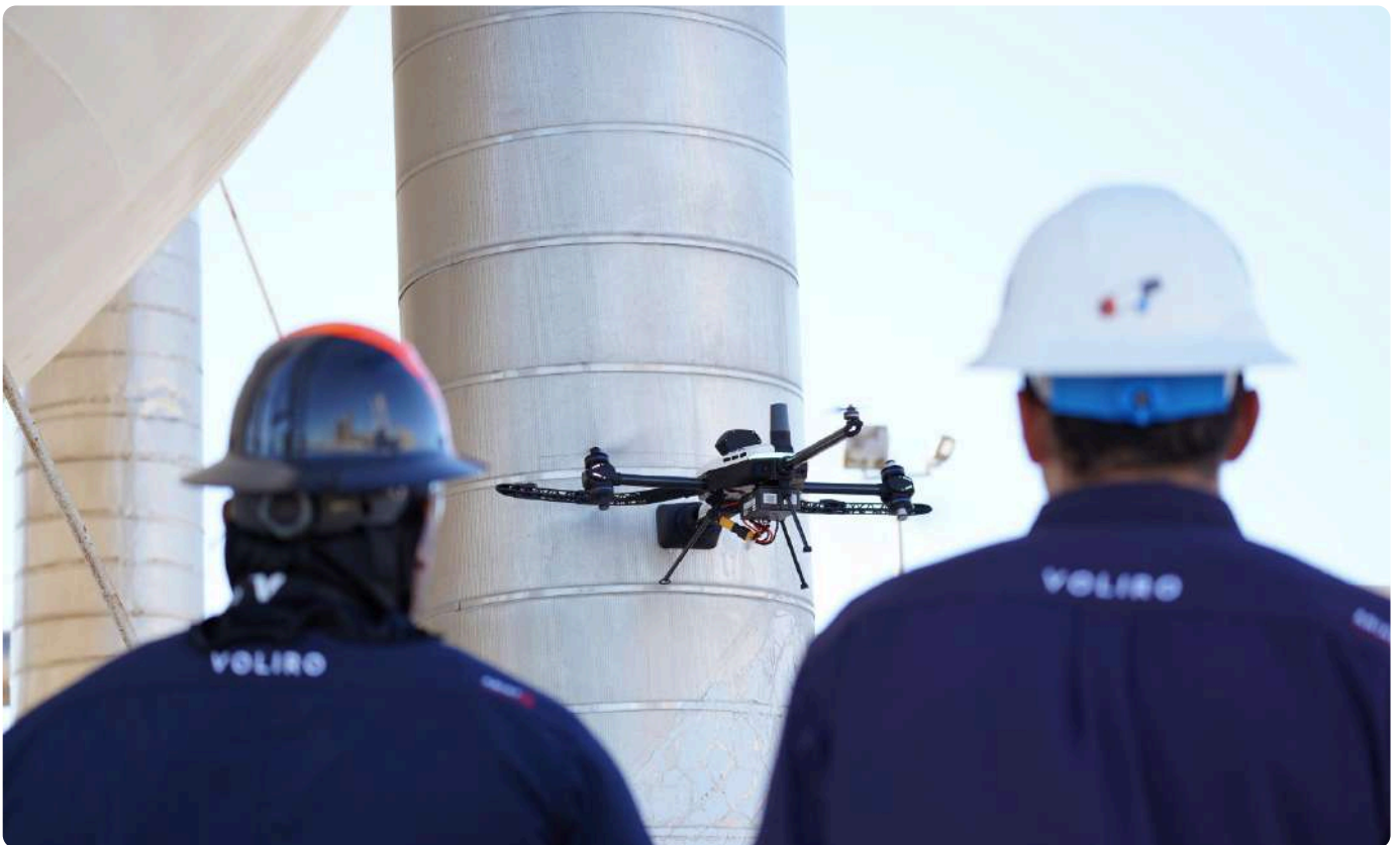
CUI inspection workflow with Voliro's drone-based Pulsed Eddy Current Sensor on insulated asset
