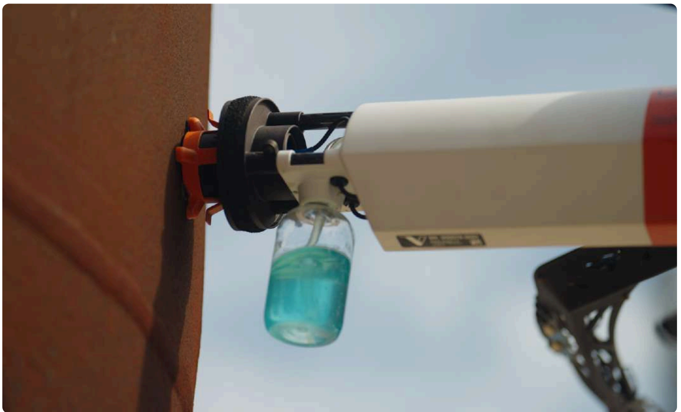
Aerial UT thickness measurement on a stack using Voliro T while asset is still in operation
