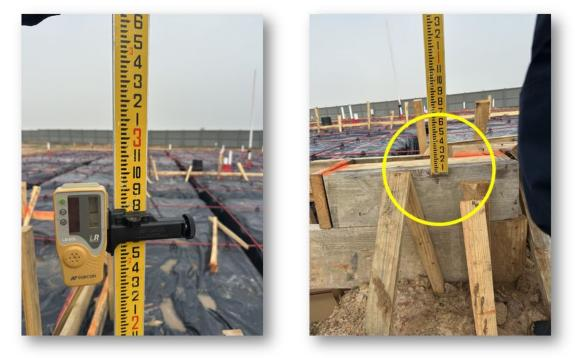
Forms were checked for level with a precision laser level instrument. Front right corner of foundation form inclosure showed 1" higher than the rest of the form boards at time of inspection. Adjust to level prior to concrete placement.
