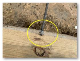
Some cathead clamps not tight to form board. Tighten all prior to concrete placement.
