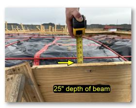
Beam depth not to 26 inches at time of inspection as prescribed in the foundation plans. Clear beams to obtain 26" of depth.
