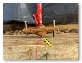
Some dead ends have exposed cable and are against the form board. Cover end and provide adequate clearance from the form board.
