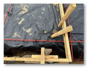
Some tears observed in the poly sheeting at the time of inspection. Tape all tears prior to concrete placement.
