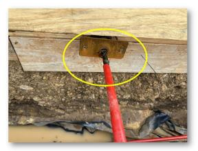
More than 1" exposed cable at some live ends. Cover with plastic or other appropriate material prior to concrete placement.
