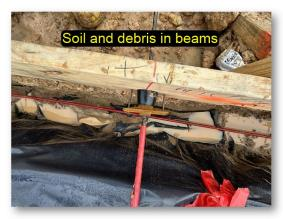
Soil and debris found to be at the bottom of some beams at the time of inspection. Clear beams prior to concrete placement.
