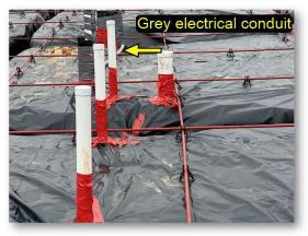
Conduit present for electric branch conductors to be routed to the island from an interior wall at future phase of construction..
