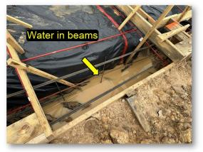
Water in beams at time of inspection. Drain all water prior to concrete placement.
