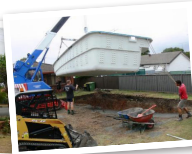
Crane used to place pool
