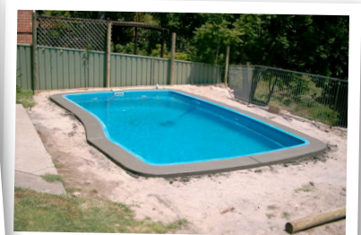
Concrete Bond Beam
