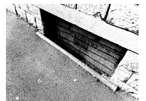
A basement access point to the cellar.
