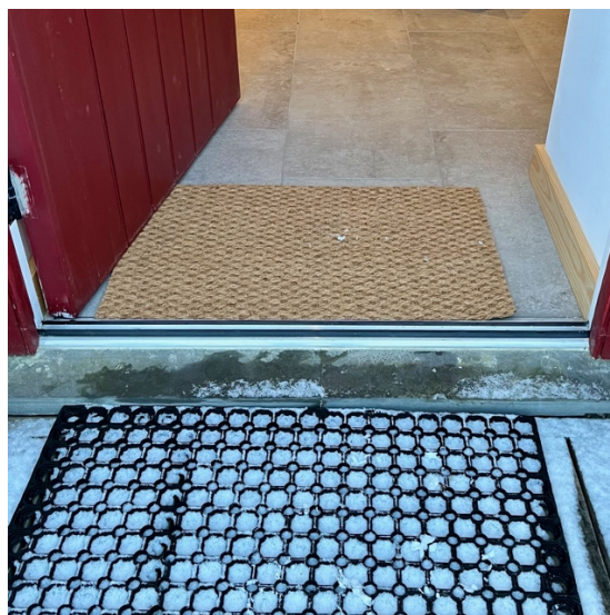
Threshold to the entrance door
