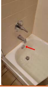
Location: BASEMENT BATHROOM
