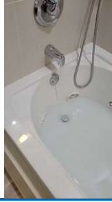
Location: MASTER BATHROOM
