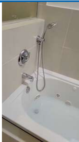
Location: MASTER BATHROOM
