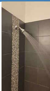
Location: HALLWAY BATHROOM
