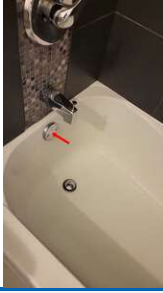
Location: HALLWAY BATHROOM
