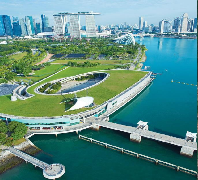
Costal Dam Marina Barrage, Singapore
