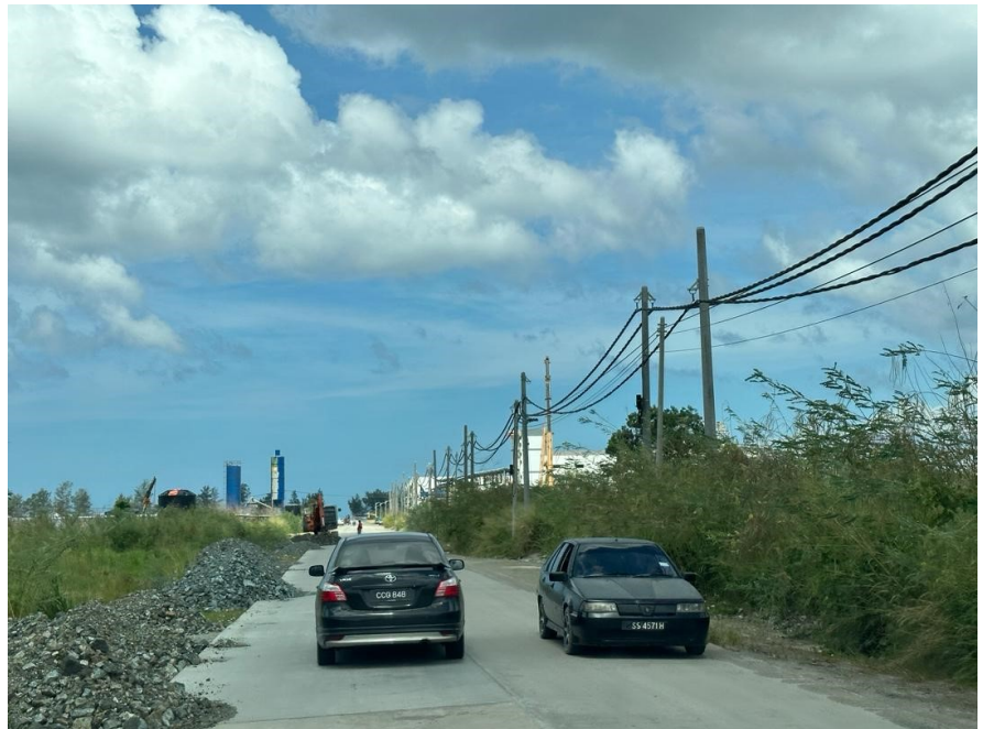
Photo 16: Road and electricity development within the project site
