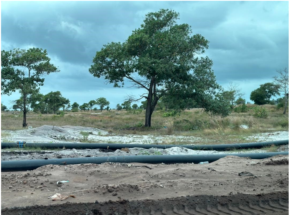
Photo 9: Raw Silica Sand is channelled to Processing Plant using 12 inches' diameter piping system.
