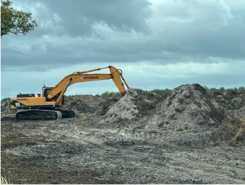
Photo 6: Ground clearance is currently carried out.
