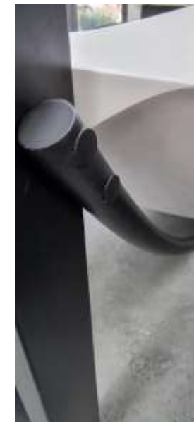
Curved brace connected to steel frame
