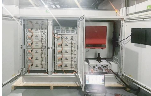
20kW / 60kWh BESS for Myanmar
