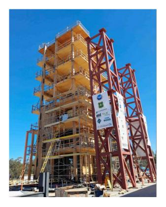
Fig. 1. TallWood is a project designed to prove that tall earthquake-protected buildings can be made of wood. Toughness of building materials, particularly under seismic activity, is extremely noteworthy in areas where earthquakes are common. Buildings in these areas are rigorously tested to prove that they can withstand these stresses. A high toughness is integral to the beams used, in the sense that these members must be able to plastically deform, and not fail under these circumstances.
