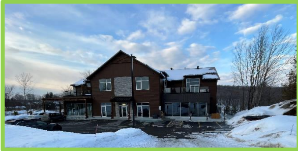
Photo 20. Primary CIP looking North at CIB.
