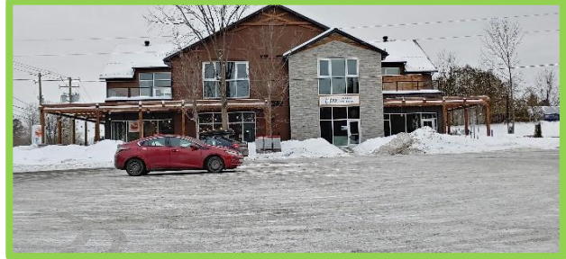
Photo 2. SSP looking East showing elevation of CIB in relation to VR and SSP.
