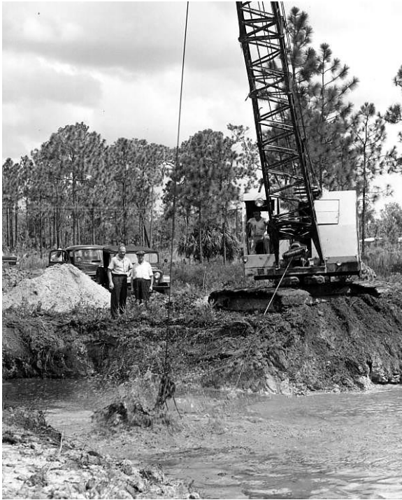
Canal being dredged across new golf course at the Port Paradise Hotel - Crystal River, Florida. Credit Florida Memory, Florida Secretary of State, State Archives.
