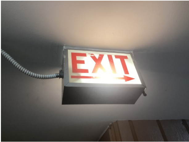
Exit signage – note finish deterioration (clubhouse shown)
