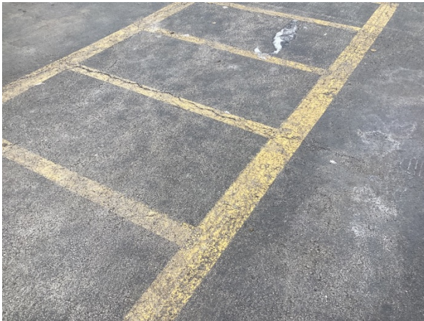
Pavement cracks
