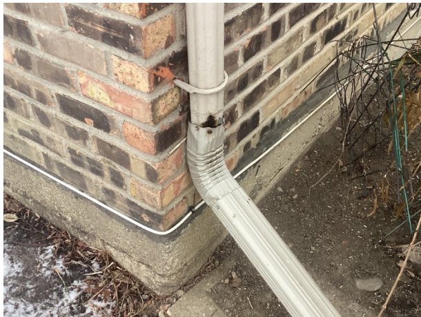
Downspout damage – note small capacity at building 13
