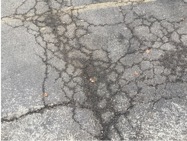
Alligator cracks
