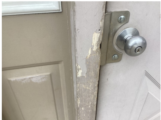
Trim finish deterioration
