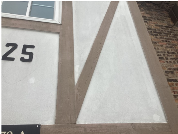
Composite hardboard siding
