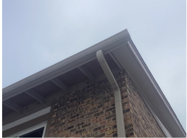
Large capacity gutters and downspouts
