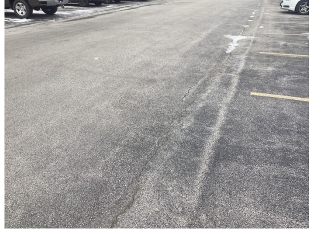
Asphalt pavement access drive overview – note cracks
