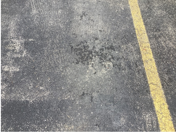
Pavement spalls
