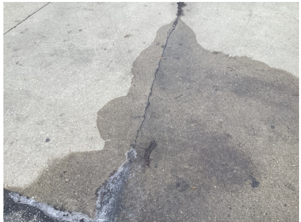
Trash pad crack
