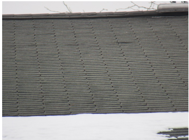
Three tab shingles – note shingle lift (remaining roof shown)
