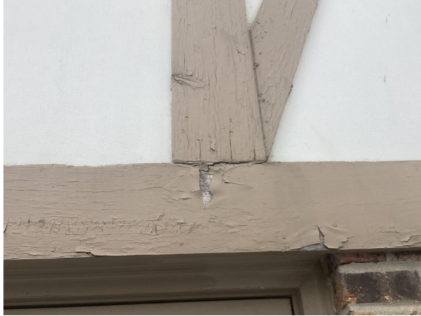
Trim finish deterioration
