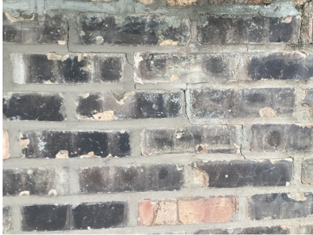
Masonry step crack
