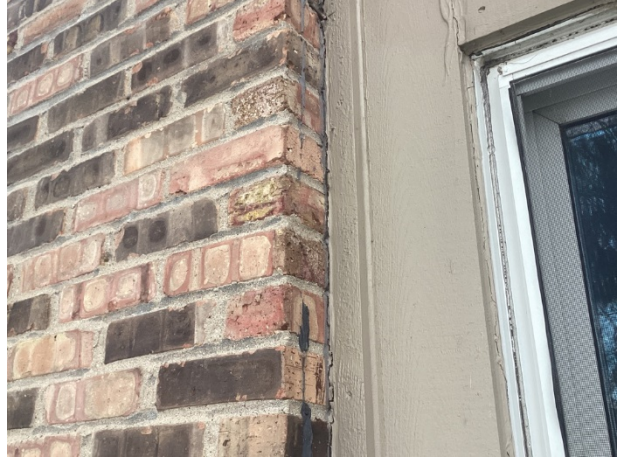
Sealant deterioration
