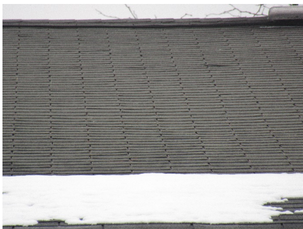
Shingle lift (building 18 shown)
