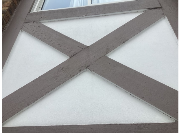
Fiber cement panel overview – note good condition
