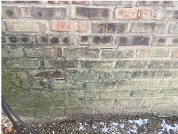
Masonry cracks
