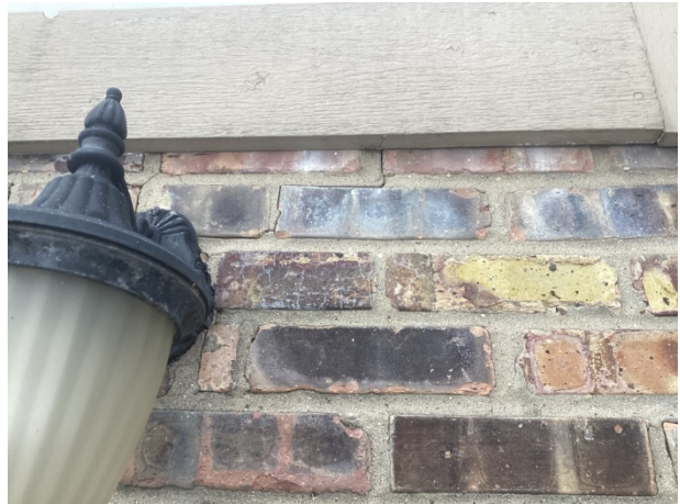
Step crack and efflorescence
