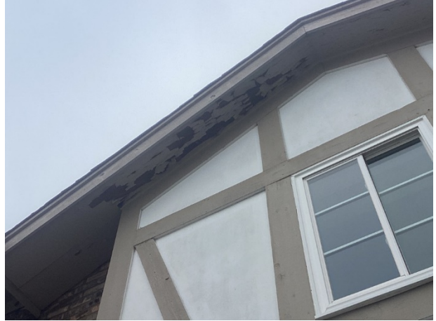
Wood soffit deterioration
