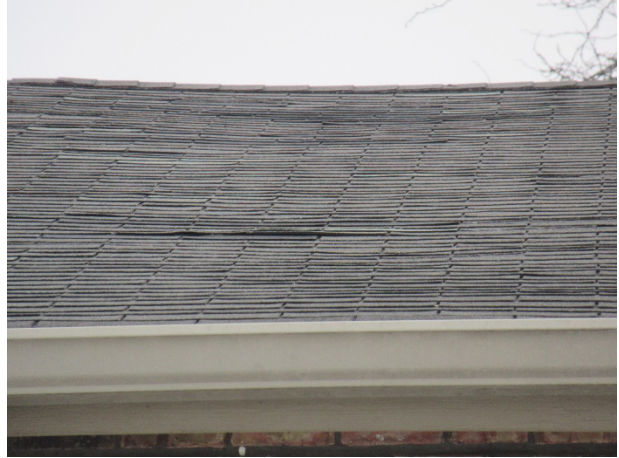
Shingle lift and shingle lift (building 16 shown)
