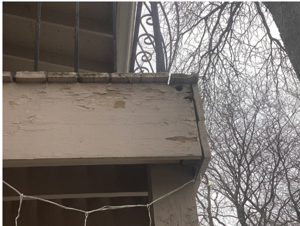
Deck board and fascia wood rot – note finish deterioration
