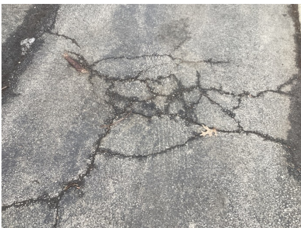
Pavement cracks
