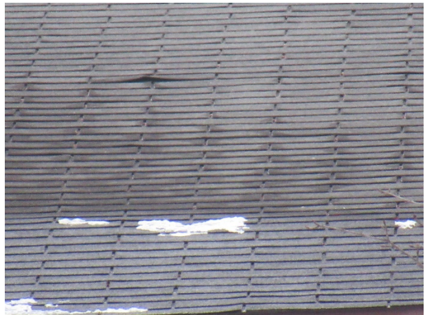
Shingle lift – note dimensional shingles (building 10 shown)
