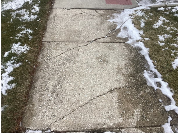
Sidewalk cracks
