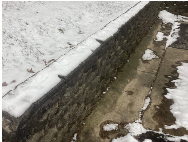
Masonry retaining wall – note organic growth
