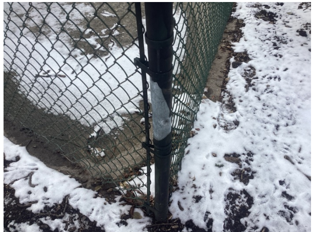
Post finish deterioration
