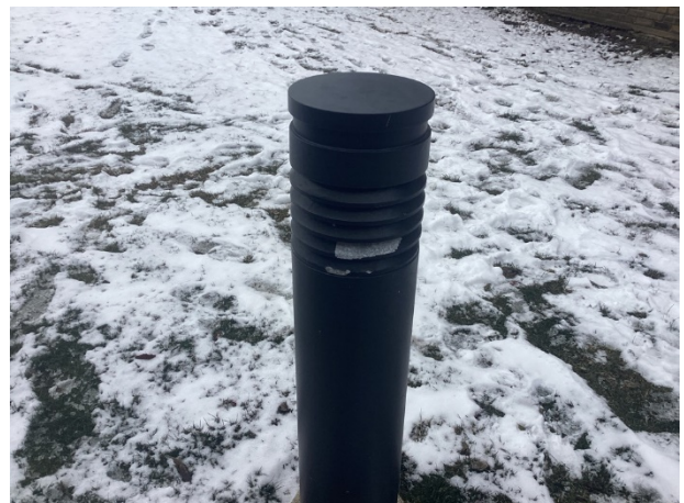
Bollard light finish deterioration
