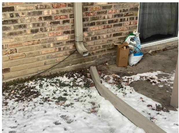
Disconnected downspout
