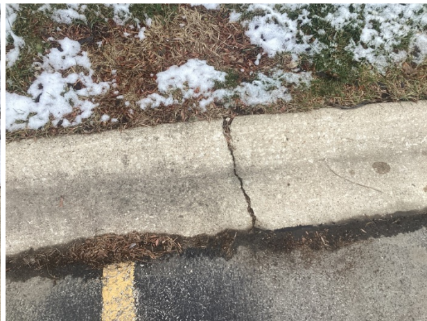
Concrete curb and gutter crack
