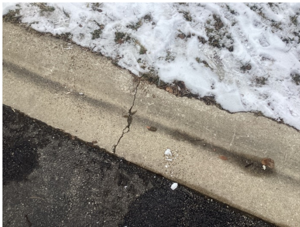
Concrete curb crack
