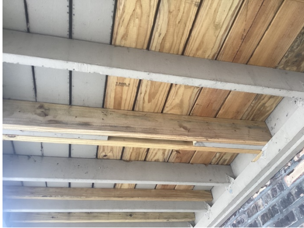
Replaced deck boards
