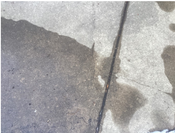
Concrete sidewalk cracks
