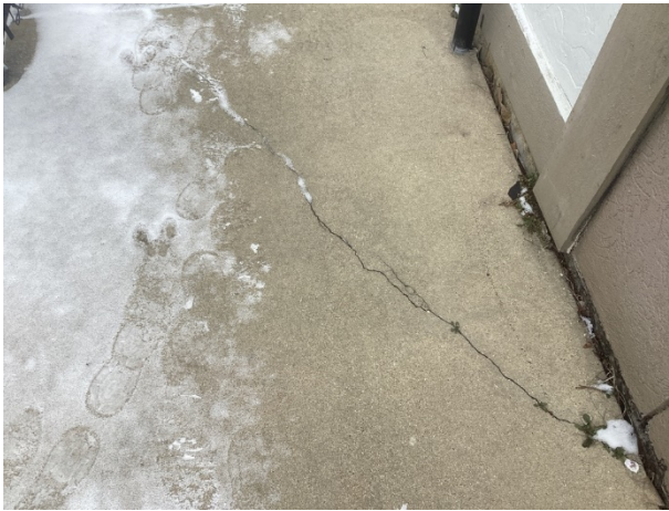
Pool deck cracks
