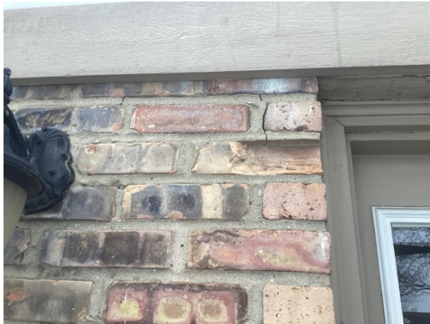
Mortar deterioration
