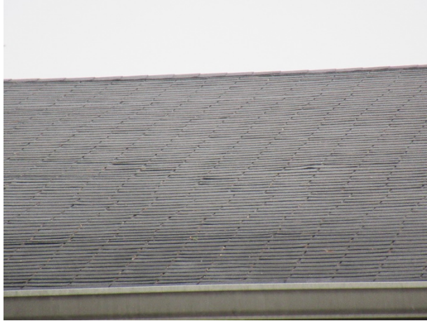
Shingle lift (building 26 shown)
