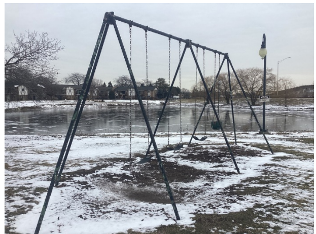
Swings – note finish deterioration
