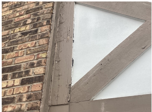
Trim finish deterioration
