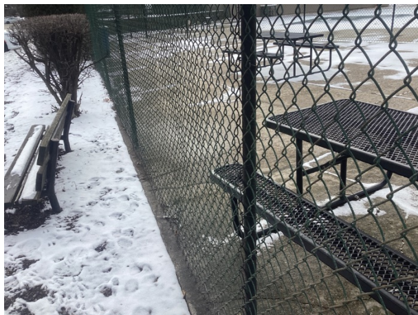
Fence warped webbing
