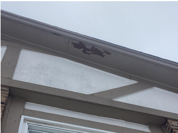
Wood soffits and fascia – note finish deterioration
