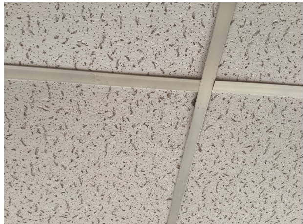
Ceiling tile damage
