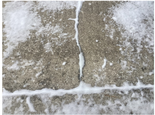
Pool deck crack
