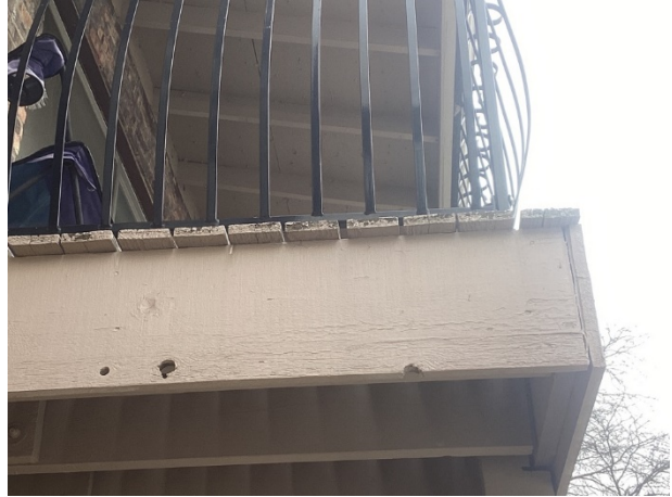
Deck board finish deterioration and organic growth
