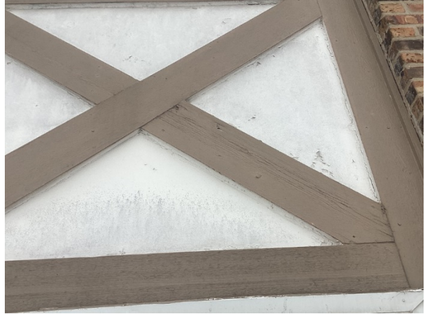
Finish deterioration and organic growth
