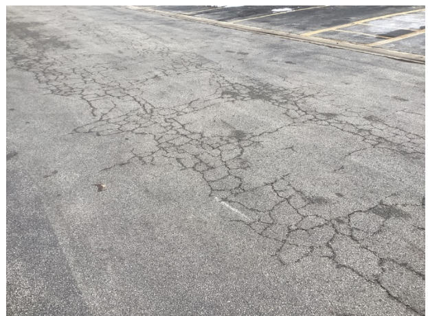
Pavement alligator cracks
