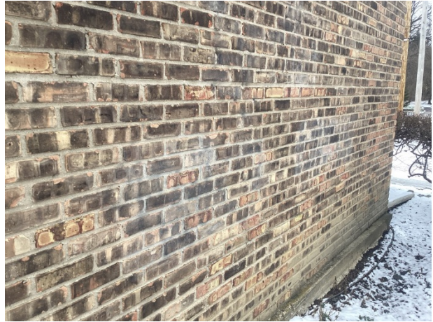
Masonry efflorescence
