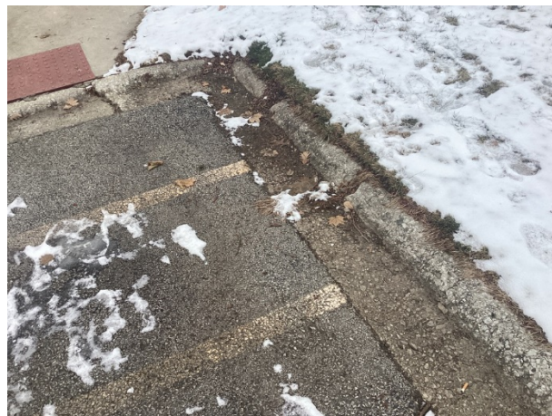
Curb settlement and damage
