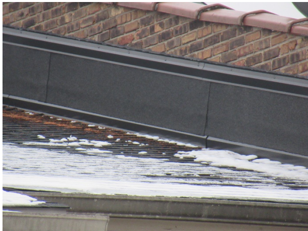
New flashing at roof parapet (recently replaced shown)
