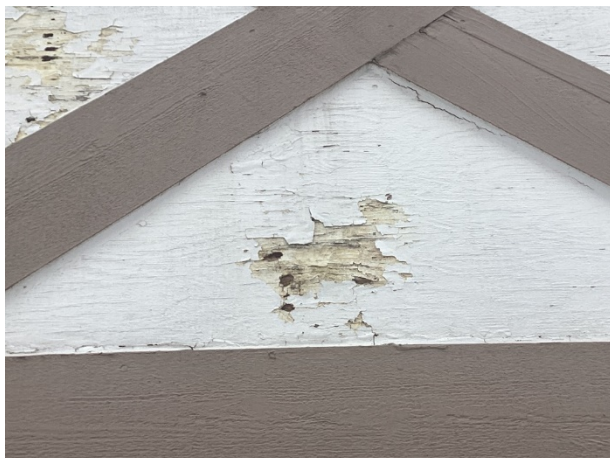
Plywood rot and finish deterioration
