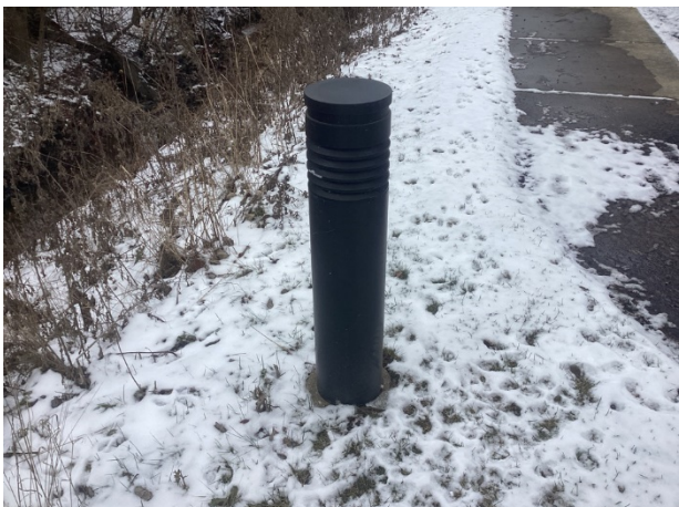
Bollard light fixture – note finish deterioration
