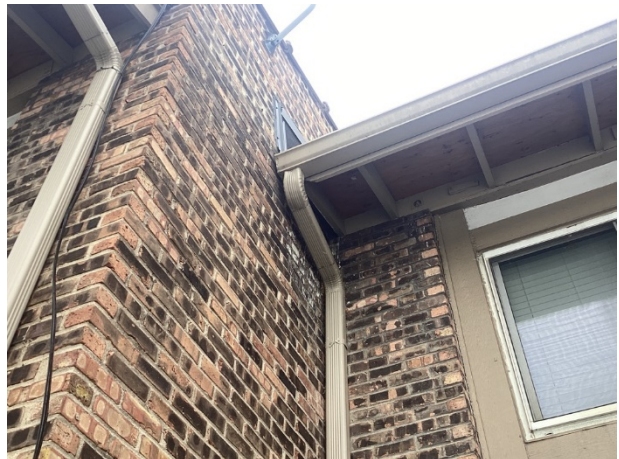
Typical gutters and downspouts
