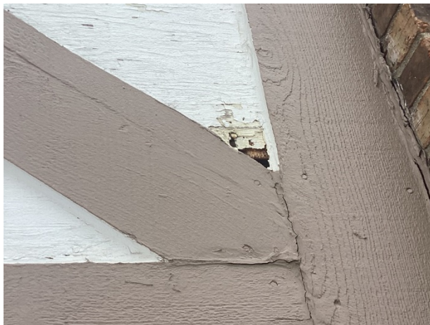
Plywood siding deterioration
