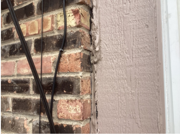
Sealant deterioration
