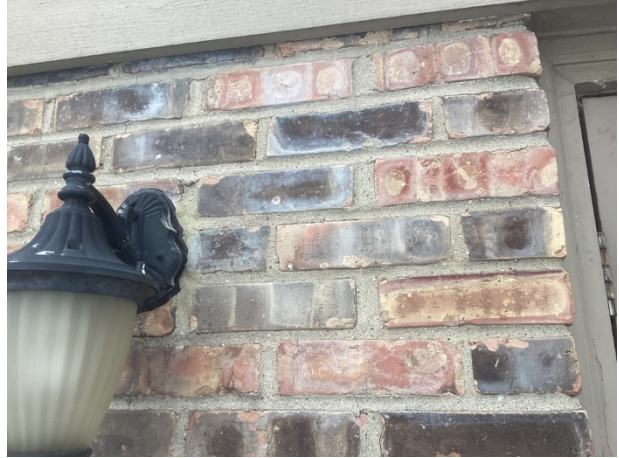
Masonry efflorescence
