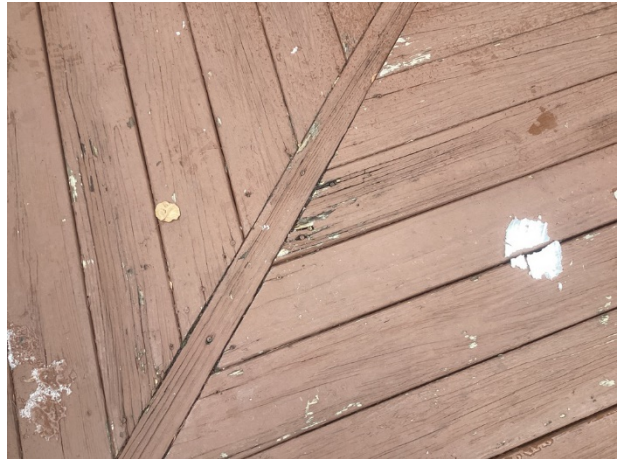
Wood rot and damage
