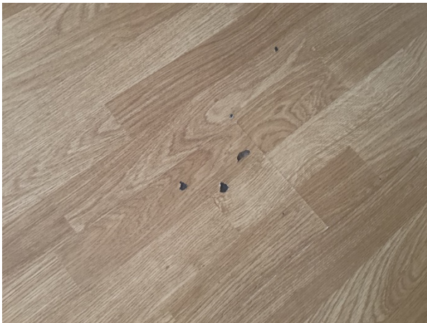
Laminate floor damage
