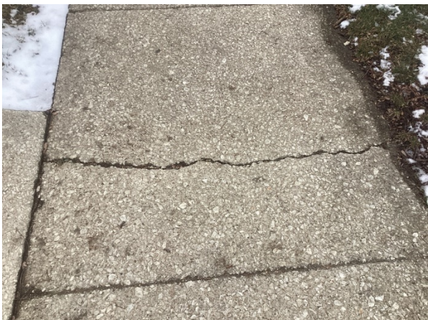
Sidewalk crack
