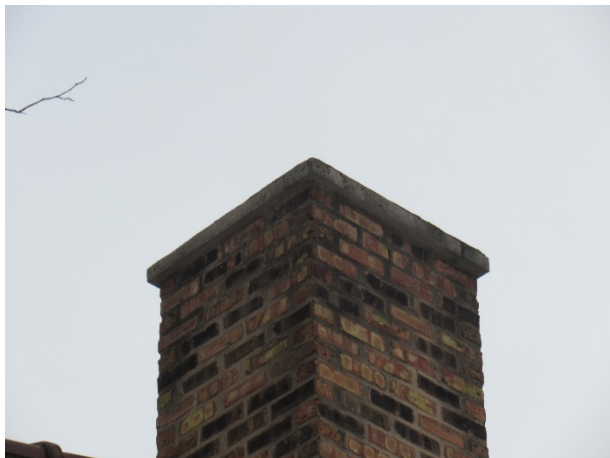
Typical chimney cap
