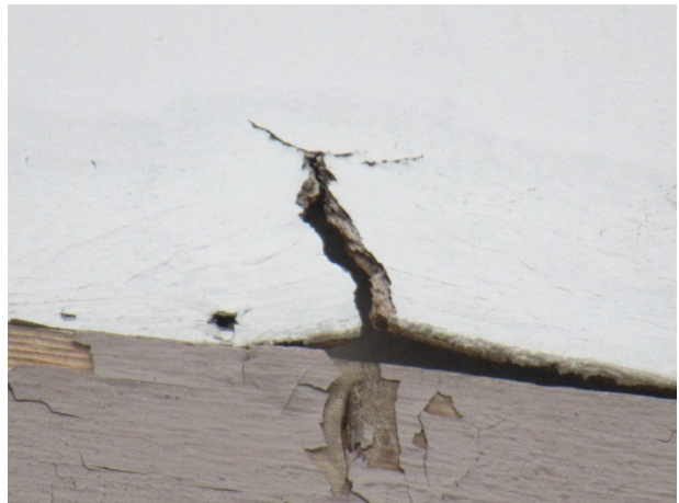
Plywood damage
