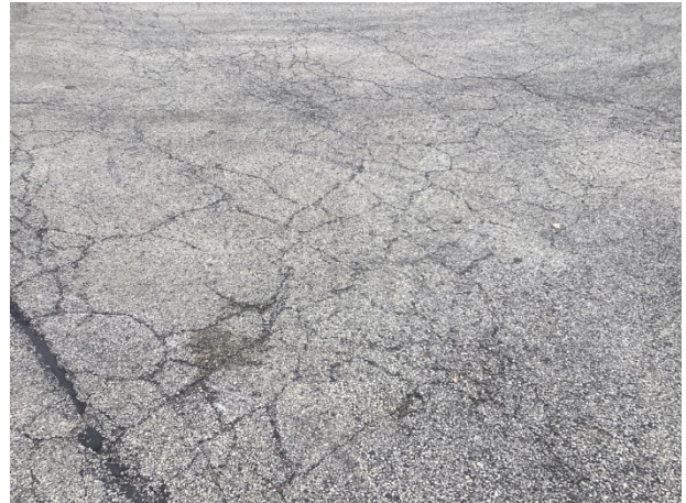
Pavement cracks
