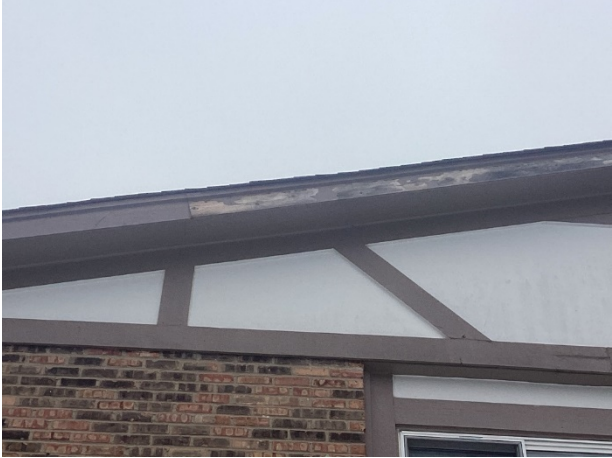
Fascia trim deterioration
