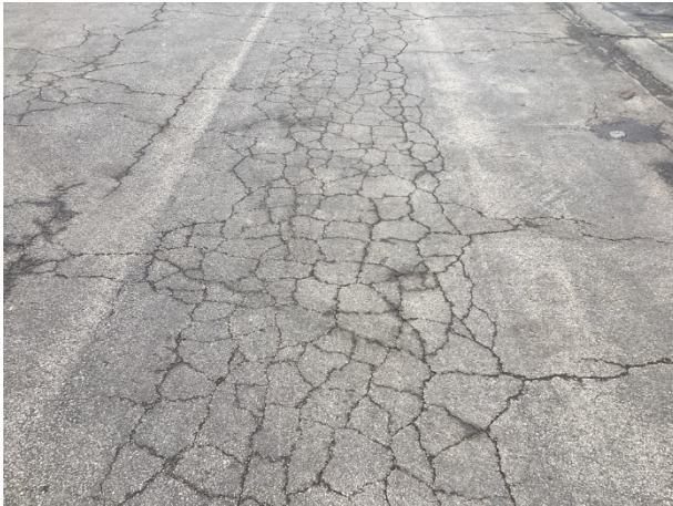
Asphalt pavement access drive overview – note alligator cracks
