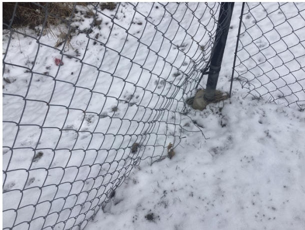
Fence warped webbing
