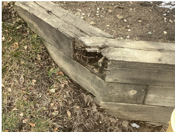
Retaining wall wood rot
