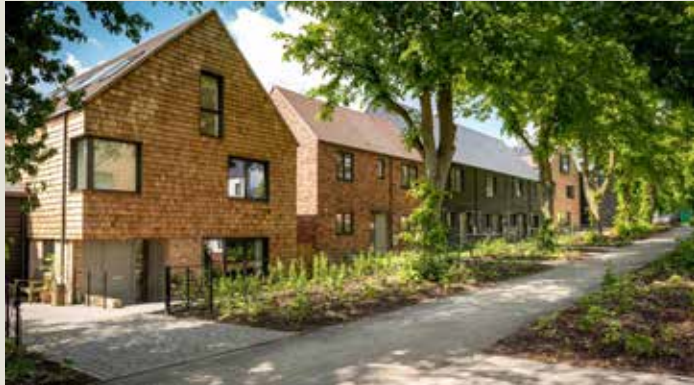
Figure 73: Low density housing enclosed within a woodland setting
