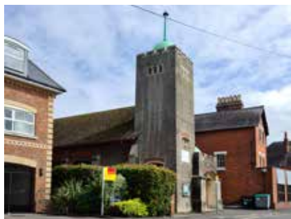
Figure 15: Methodist Church, Listed Grade II
