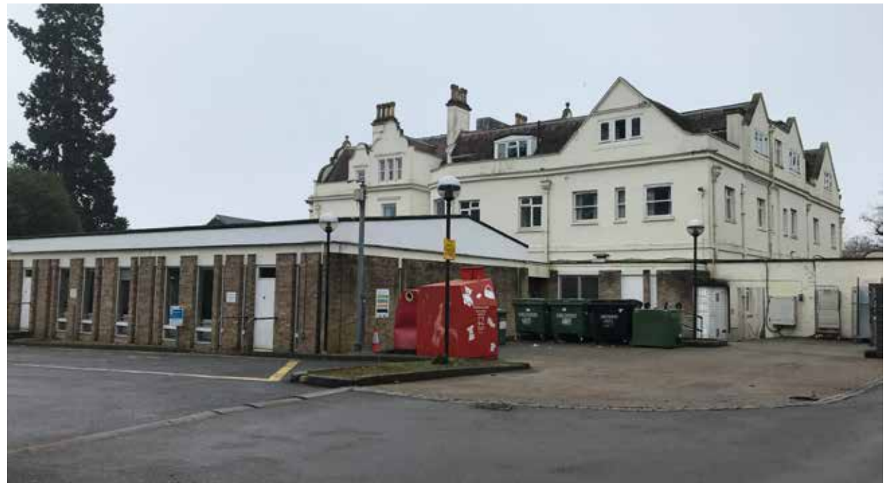
Figure 68: Eastern elevation of Kingswood
