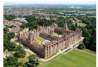
Main University Building
