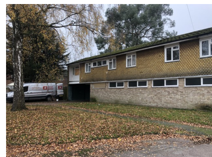
Property with Boarded Windows
