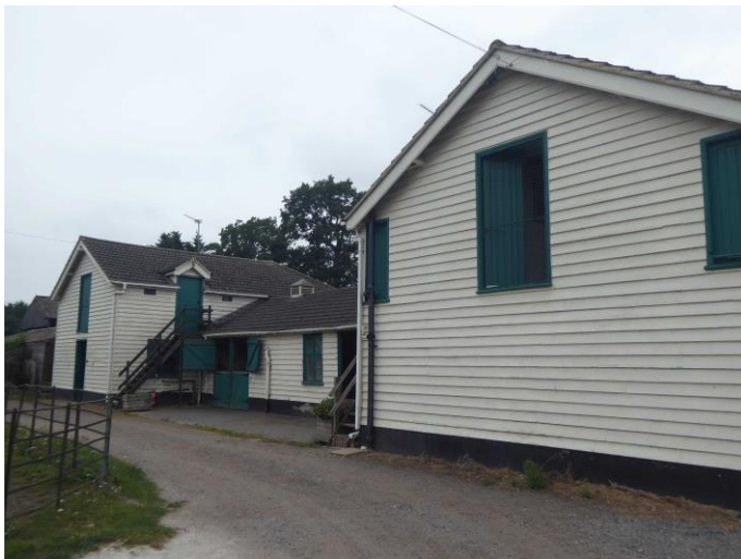
The stables looking west.
