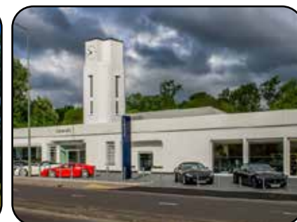
15. Tower Garage, Listed Grade II
