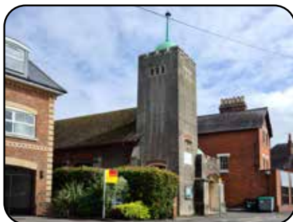
2. Methodist church, Listed Grade II
