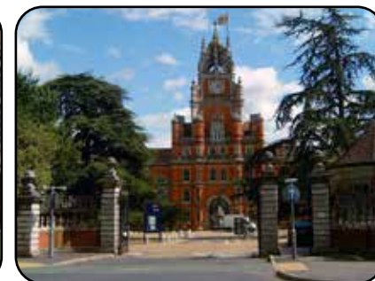
5. Royal Holloway Entrance Gates, Listed Grade II
