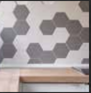
DADO CERAMIC TILES 600 MM ABOVE THE COUNTER
