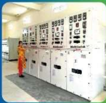
11 KV HT PANEL, HAL
